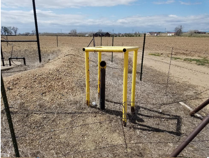
Photo 5. Unmarked riser with no LO/TO
