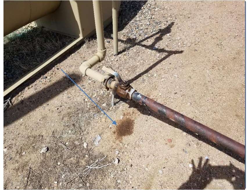
Photo 3. Stained soil near heated treater under valve
