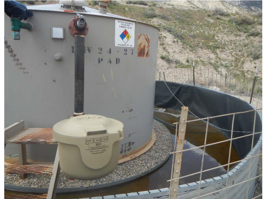
80 bbl PW tank with loadout inside SPCC. Water is apparent precipitation w no sheen or odor.
