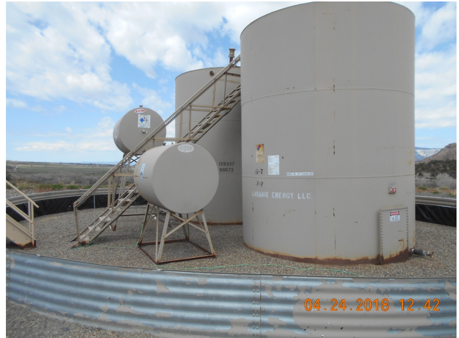
Condensate tank battery
