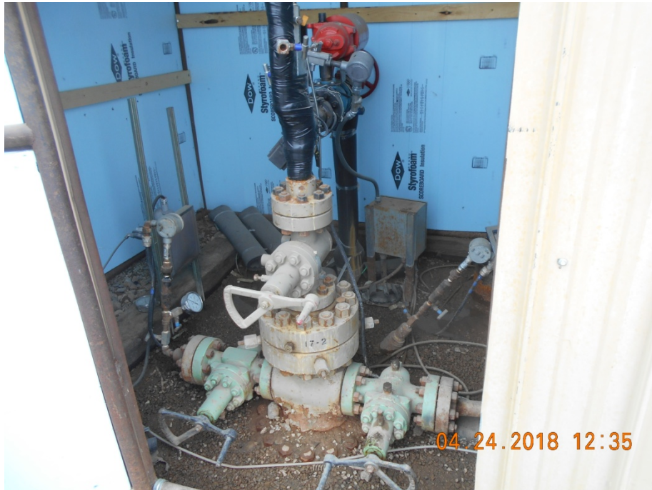
Injection wellhead inside housing
