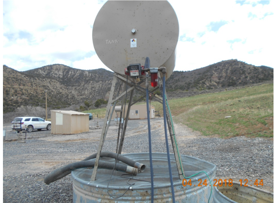
Secondary containment of fuel tank.
