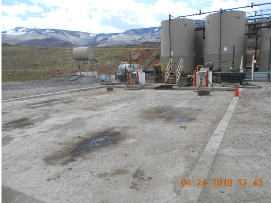
Produced water tank battery with offload stations
