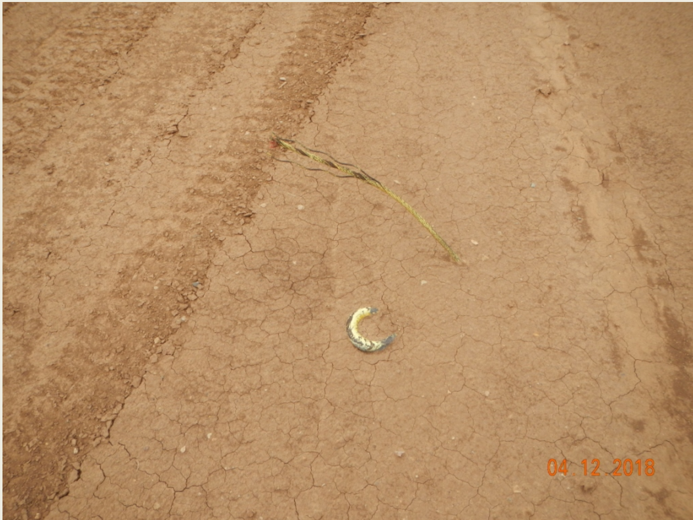
Photo 6. Guy line anchor not marked.
