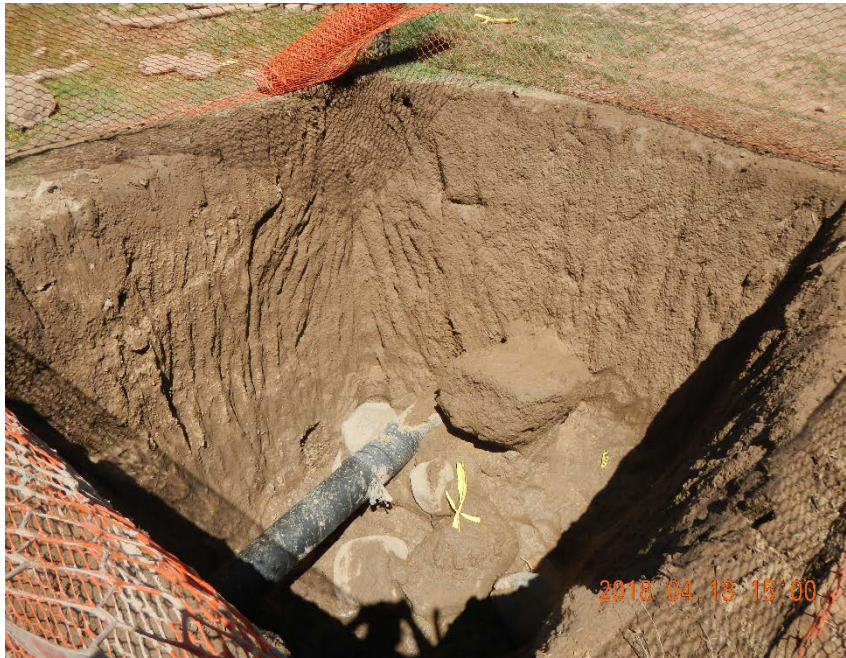
Excavation with hydrovac to expose the pipeline. The soil is composed of almost pure clay.
