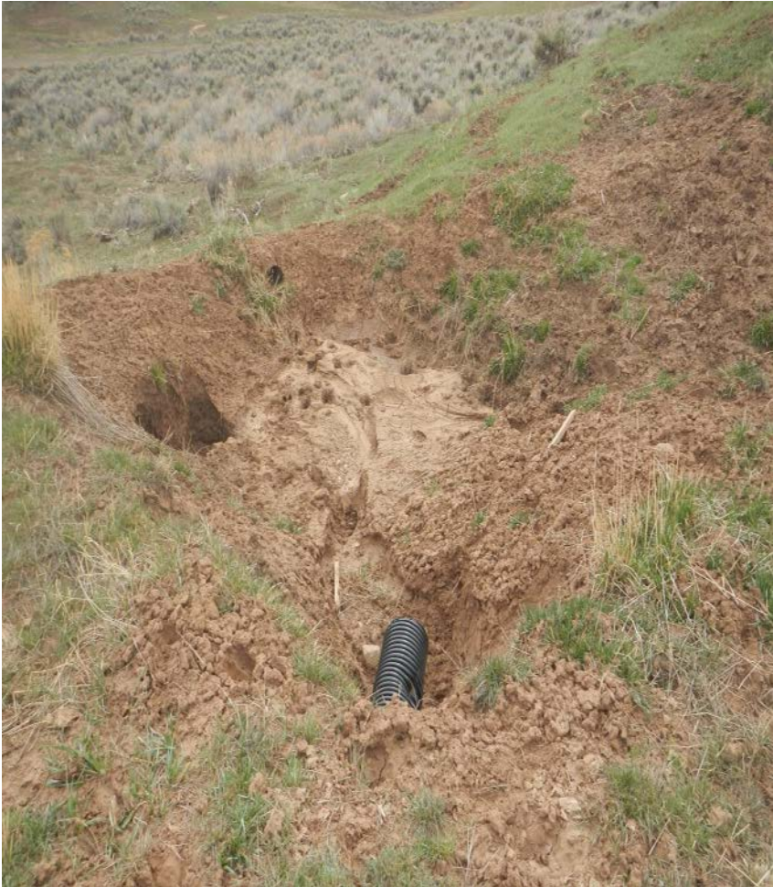
Photo#5: Sediment traps & drains leading to & at base of Fill slope have failed.
