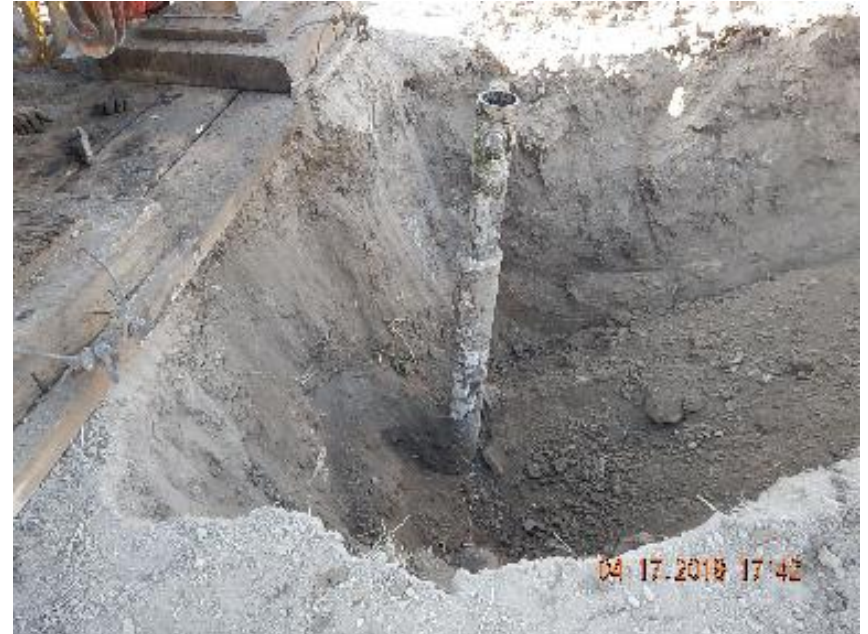
Photo 4: Casing excavation work.
