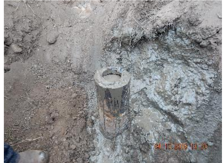
Photo 6: Casing cut off 4' below grade.
