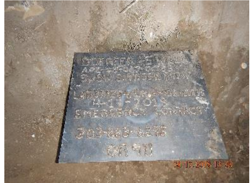
Photo 8: Installed plug and abandon marker.
