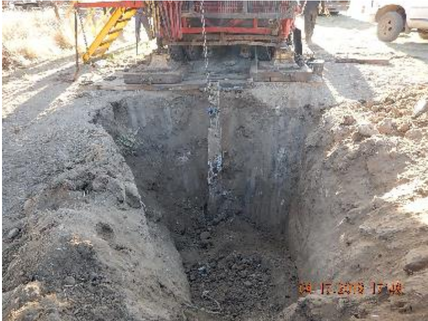
Photo 5: Completed casing excavation.
