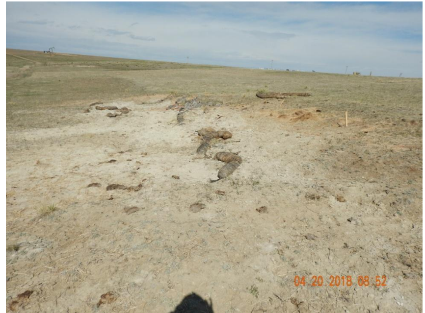
Photo 6. Photo taken from the northern well location on April 20, 2018, facing West. Appears the Operator has installed BMPs to control erosion but all the BMPs have been damaged due to cattle. Operator may need to coordinate with the surface owner to exclude cattle around the oil and gas location.
