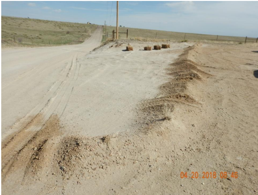
Photo 5. Photo taken from the southern battery location on April 20, 2018, facing North. Photo illustrates berm BMP has been damaged due to vehicle traffic and is not in proper functioning condition.
