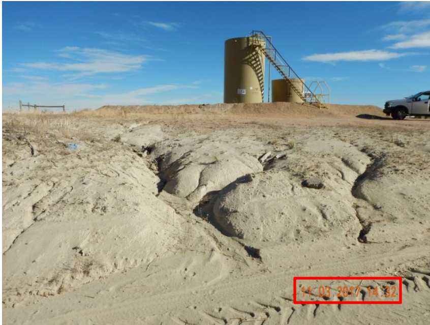
Photo 1. Photo taken from the northwest battery location on November 3, 2017, facing East. Gully erosion evident and no observed BMPs have been implemented to control and manage stormwater erosion along any portion of the location.
