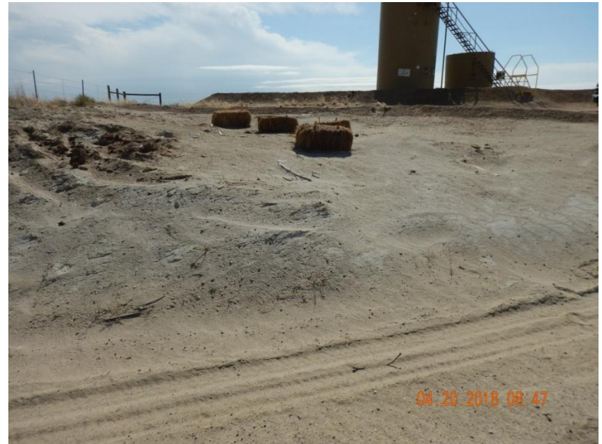
Photo 2. Photo taken from the northwest battery location on April 20, 2018, facing East. Operator made repairs to the gully erosion and installed BMPs (i.e straw bales and berm). Berm BMP has been damaged due to vehicle traffic and is not in proper functioning condition.
