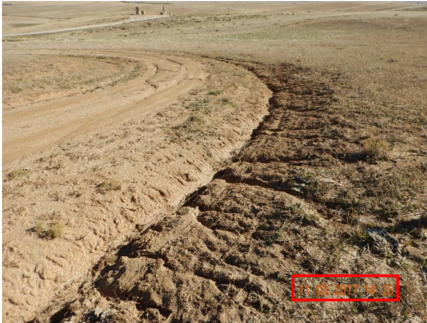
Photo 7. Photo taken from a portion of the access road on November 3, 2017, facing South. Rill erosion forming into gully erosion is evident along the access road. Operator needs to repair erosion and install sufficient BMPs.
