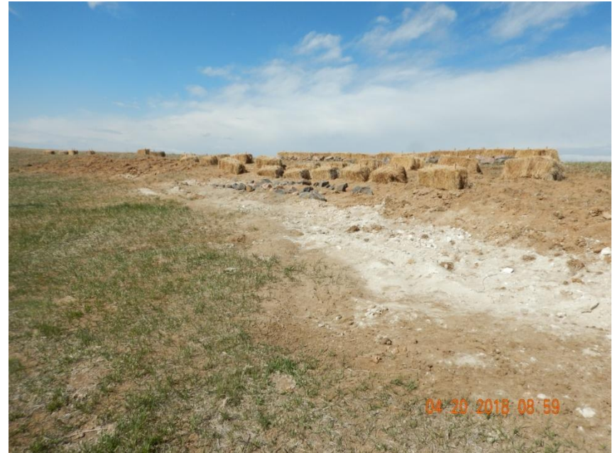
Photo 6. Photo taken from the western well pad location on April 20, 2018, facing West. Operator made repairs to the gully erosion and installed additional BMPs (i.e, more rip-rap, straw bales and surface roughening).
