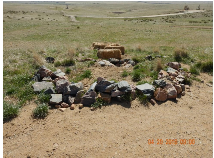
Photo 2. Photo taken from the northeast well pad on April 20, 2018, facing East. Operator made repairs to the gully erosion and installed additional BMPs (i.e., more rip-rap and straw bales).
