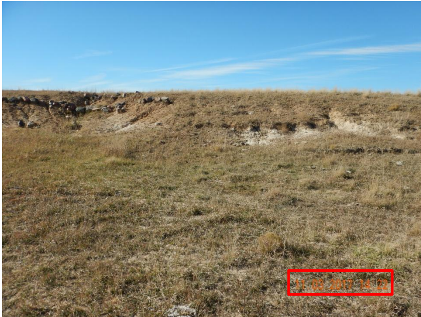
Photo 5. Photo taken from the western well pad location on November 3, 2017, facing West. Appears stormwater run-on onto the location is causing gully erosion along the western cut slope which is causing degradation to the location. Operator needs to repair gully erosion and install sufficient BMPs.
