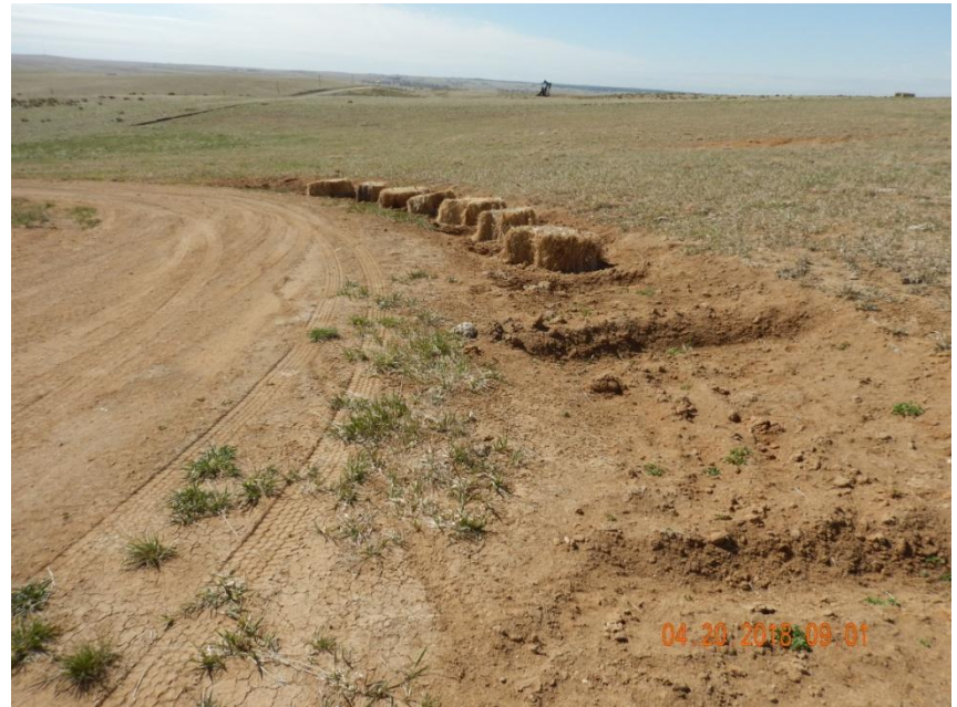
Photo 8. Photo taken from a portion of the access road on April 20, 2018, facing South. Operator made repairs and installed BMPs (i.e, straw bales and surface roughening).
