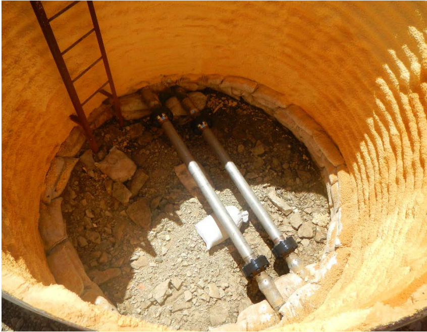
Can 41 with repaired piping
