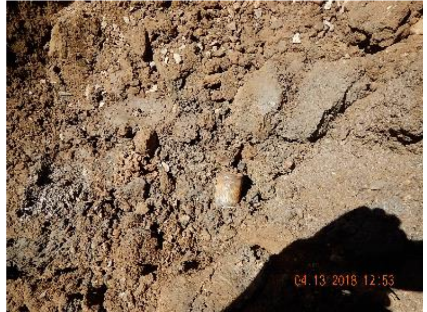
Photo 4: 2" steel flow line to tank plugged with 2" steel bull plug.
