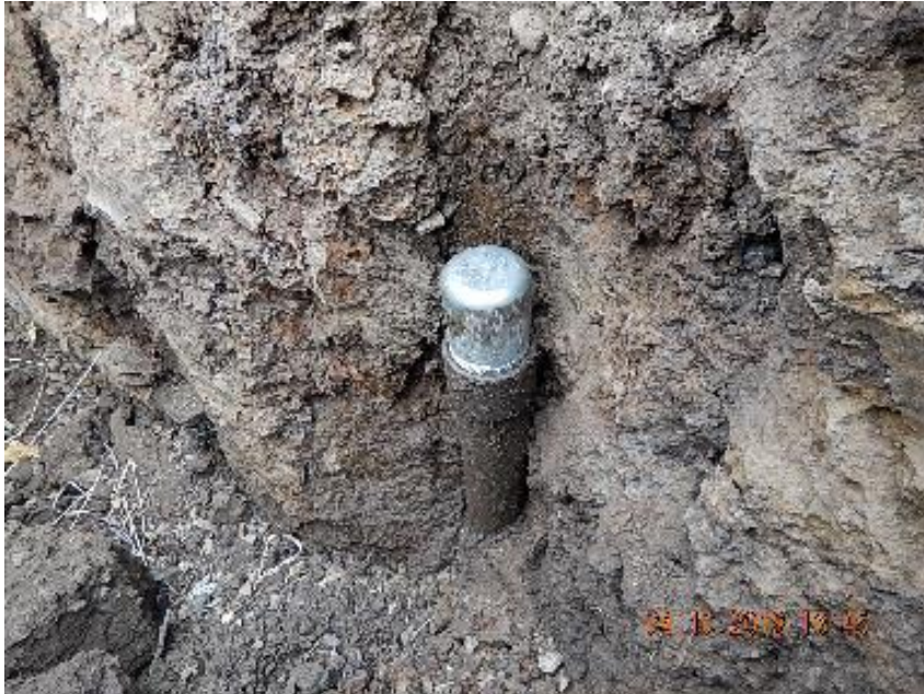
Photo 3: 2" steel flow line at production tank riser plugged on tank side with 2" steel bull plug.
