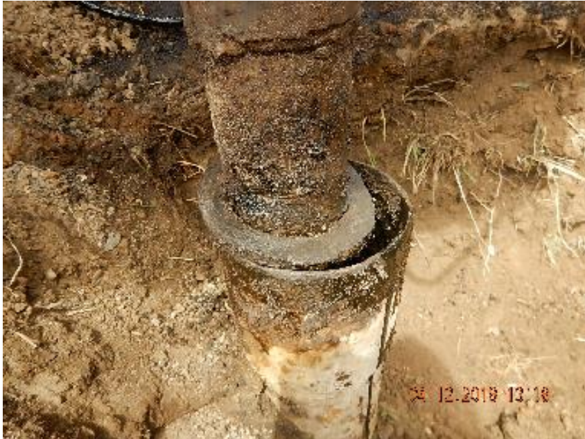
Photo 3: Separated ring at the top of casing.
