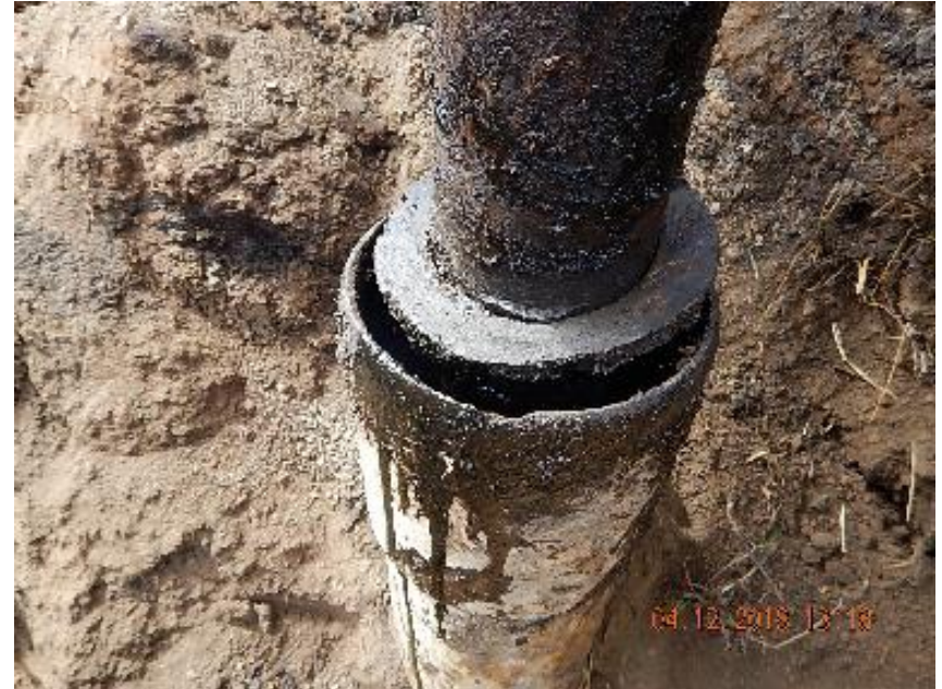
Photo 4: Worked ring up to allow free returns while pumping cement.
