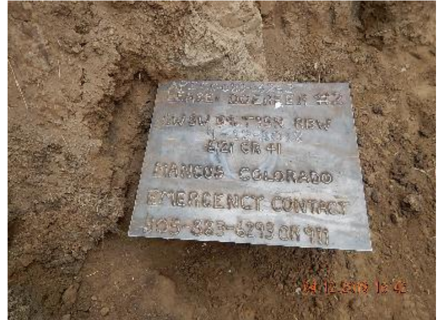
Photo 8: Plug and abandon marker welded onto casing.
