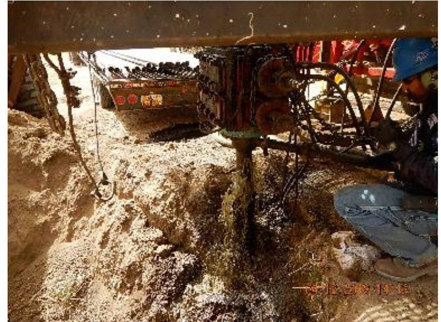
Photo 6: Returns out of top of casing into excavated hole. Fluids collected and vacuum truck removed them.
