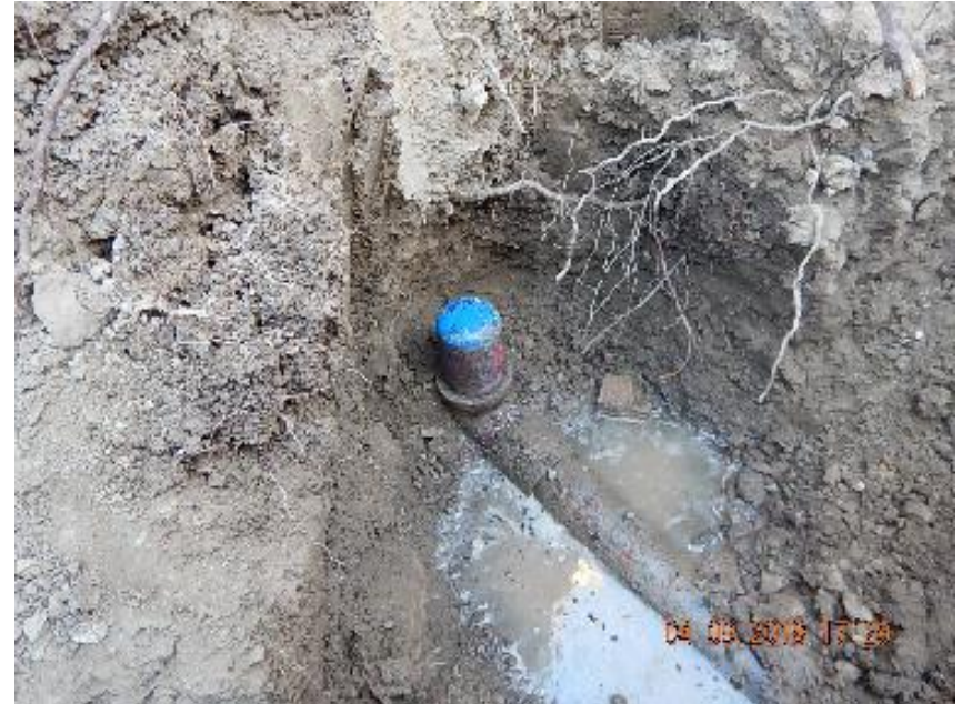
Photo 10: Plugged 2" flow line with 2" bull plug.
