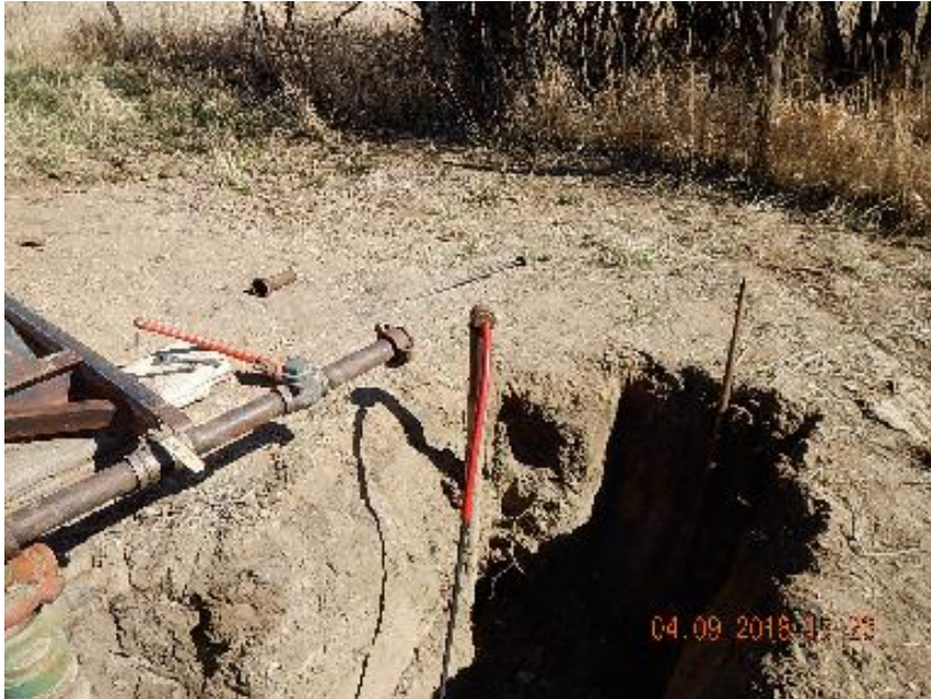
Photo 9: Excavated flow line riser and flush line tied into riser.
