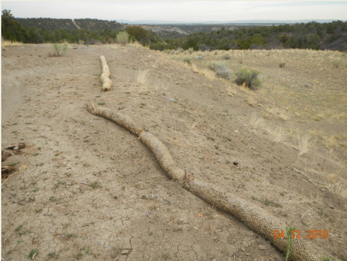
Photo 3. Close-up view of wattles and recently repaired erosional channel in the southern project area.
