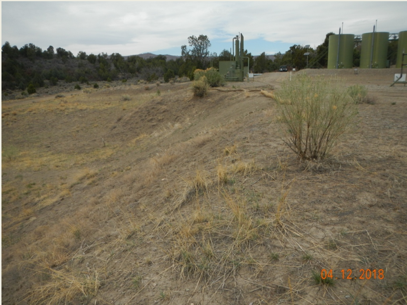
Photo 2. View of the southern portion of the project area from the southeastern corner facing westward. Temporary stormwater controls are installed along the southern edge of the working surface. This will need careful monitoring and maintenance or more permanent stormwater controls if erosion is occurring.
