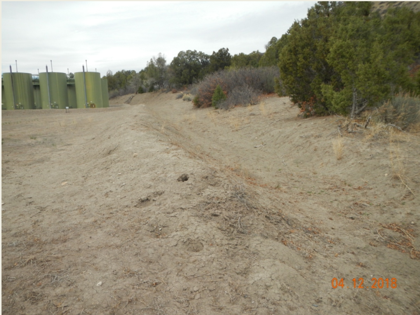
Photo 4. View of the northern project area from the northeastern corner facing westward. Berms do not appear properly stabilized and diversion channel is full of sediment.
