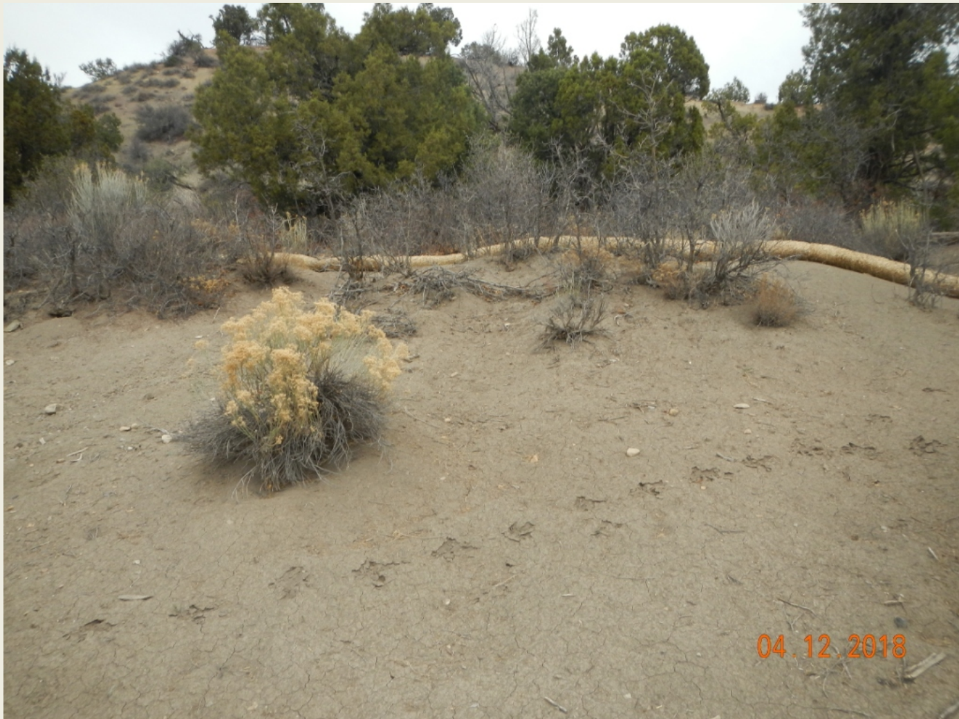
Photo 6. View of run-on controls installed in the northern portion of the project area. Cut-slope (downstream of wattles) is not stabilized.
