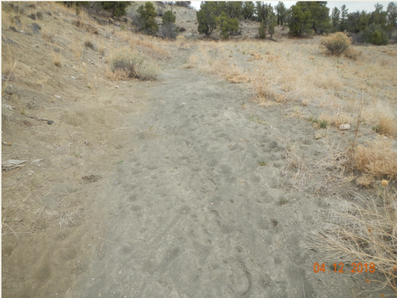
Photo 5. View of western diversion that is filled with sediment and needs maintenance.
