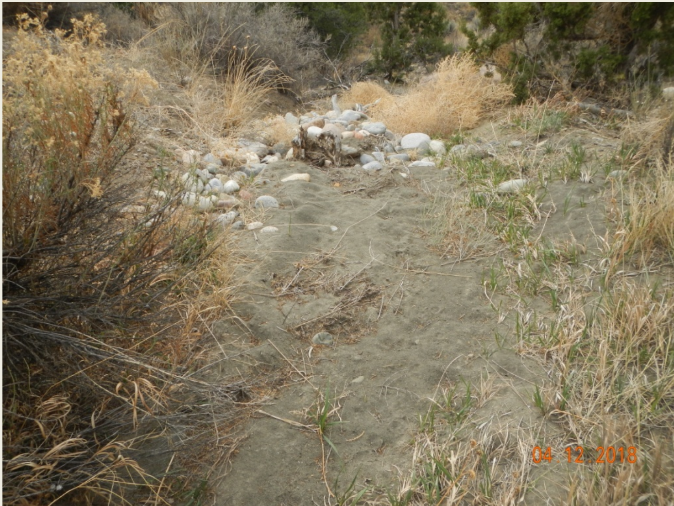
Photo 6. View of cobble run-down that is full of sediment and needs maintenance. Does not appear sufficient for sediment control.
