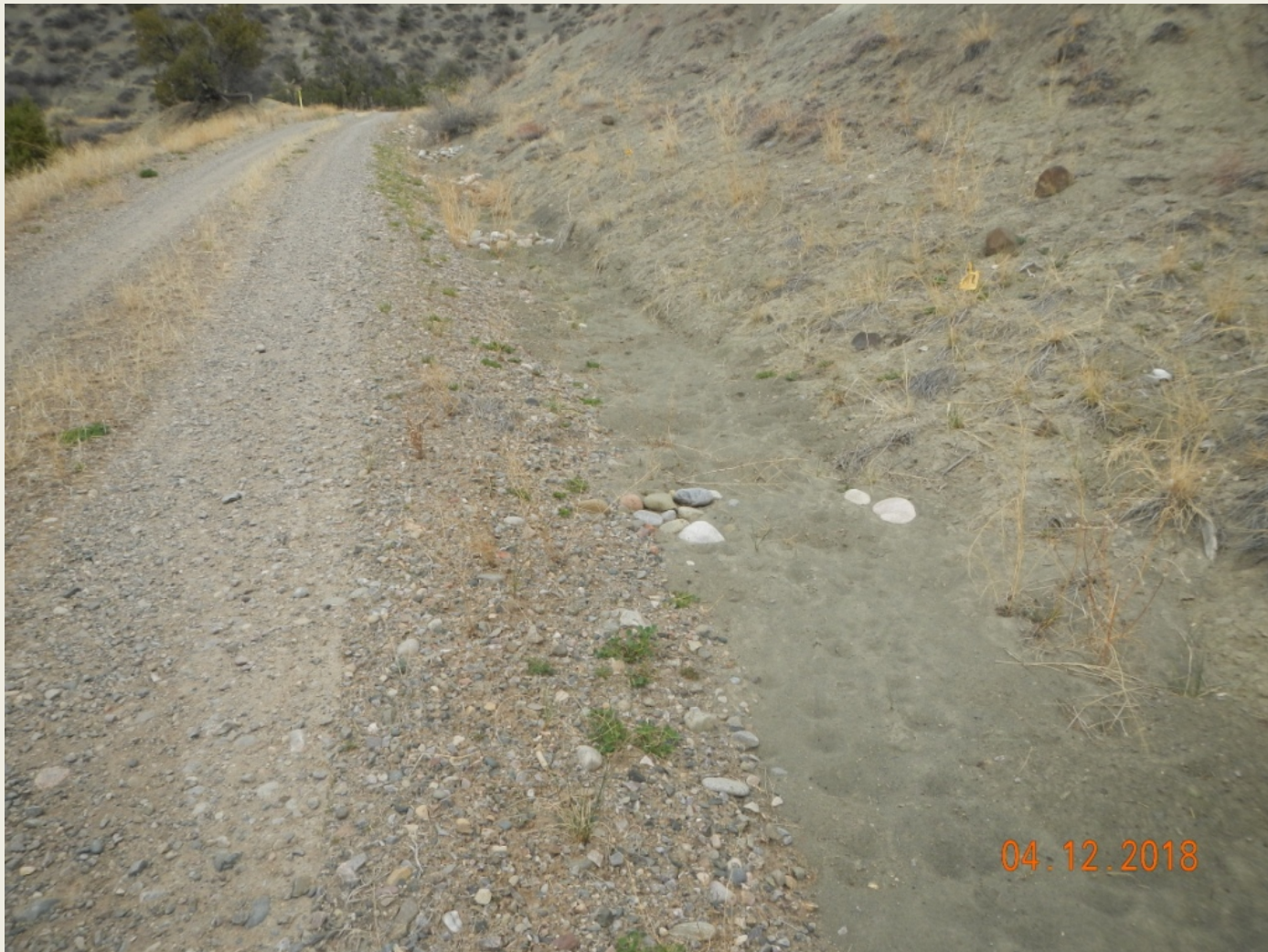
Photo 10. View of cobble check dams along the access road, full of sediment needing maintenance/repair.
