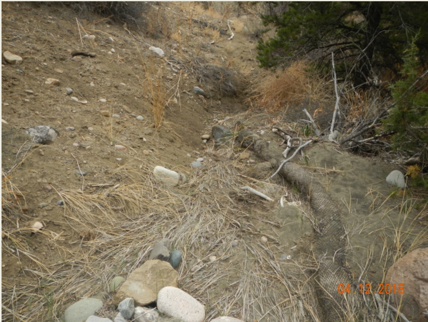
Photo 7. View of wattle failure and erosion occurring in the southwestern portion of the project area.
