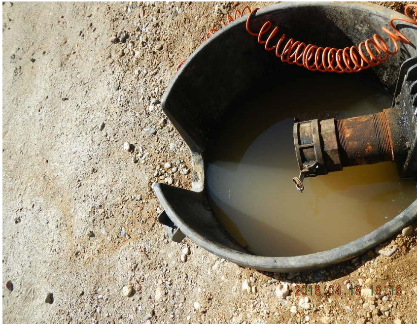
Produced water load out catchment containment ½ inch from over flowing
