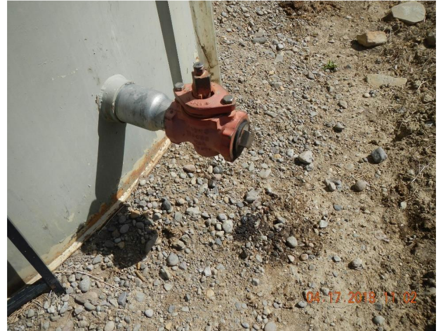
Stained soil beneath load out valve.
