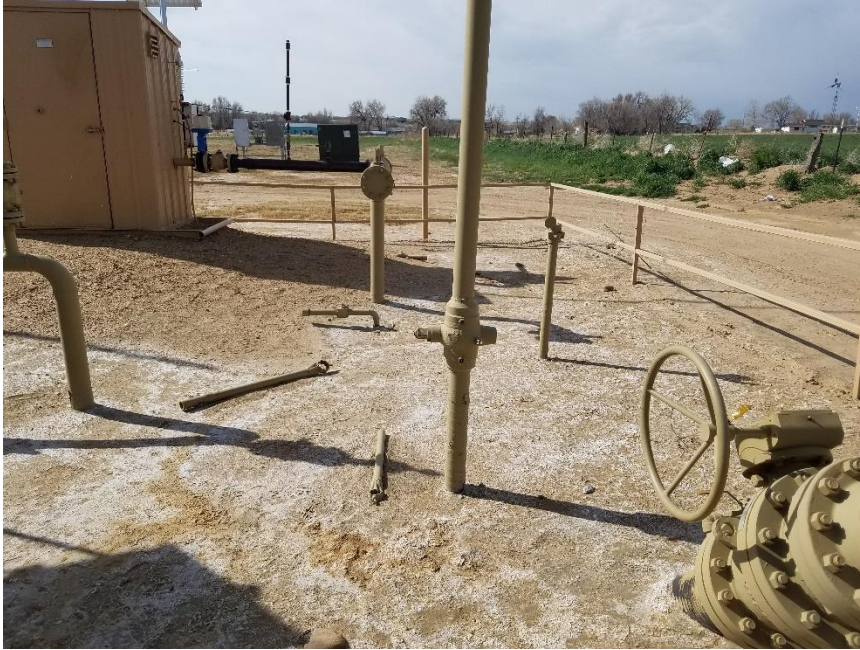
Photo 3. Unmarked risers
