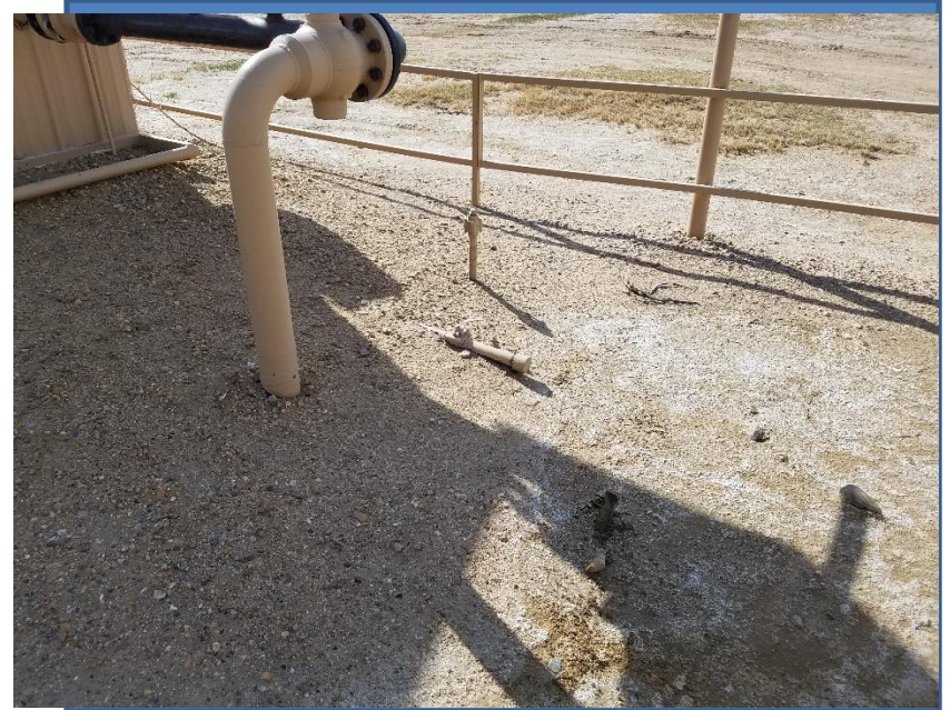
Photo 4. Unmarked risers
