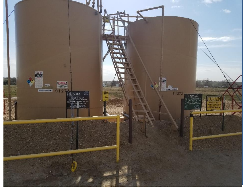
Photo 2. Tank battery
