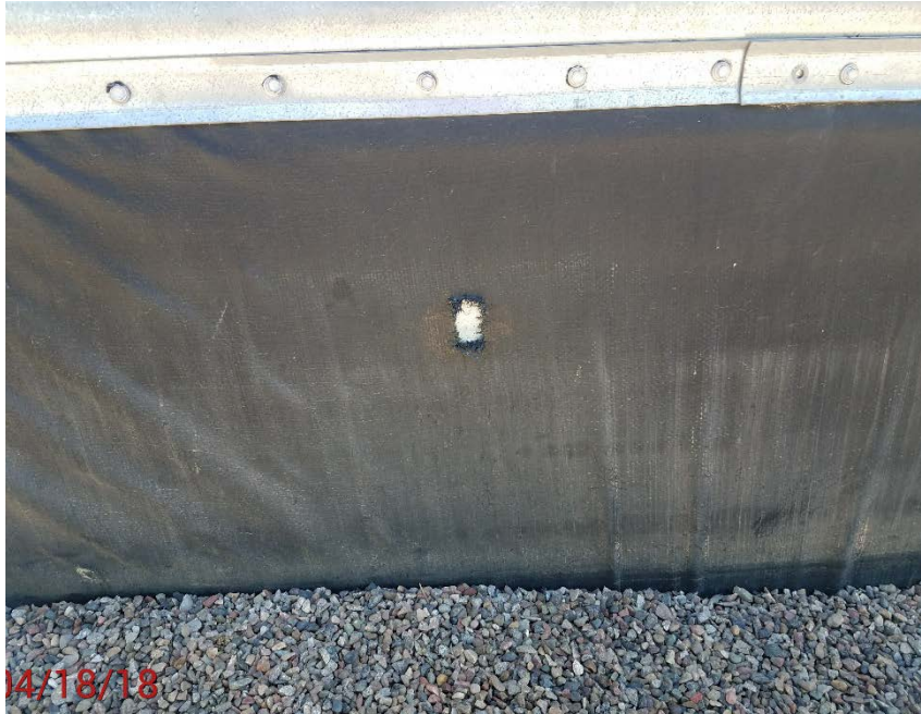
Location photo # 3, hole in containment
