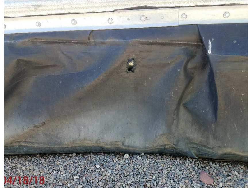
Location Photo # 4, hole containment
