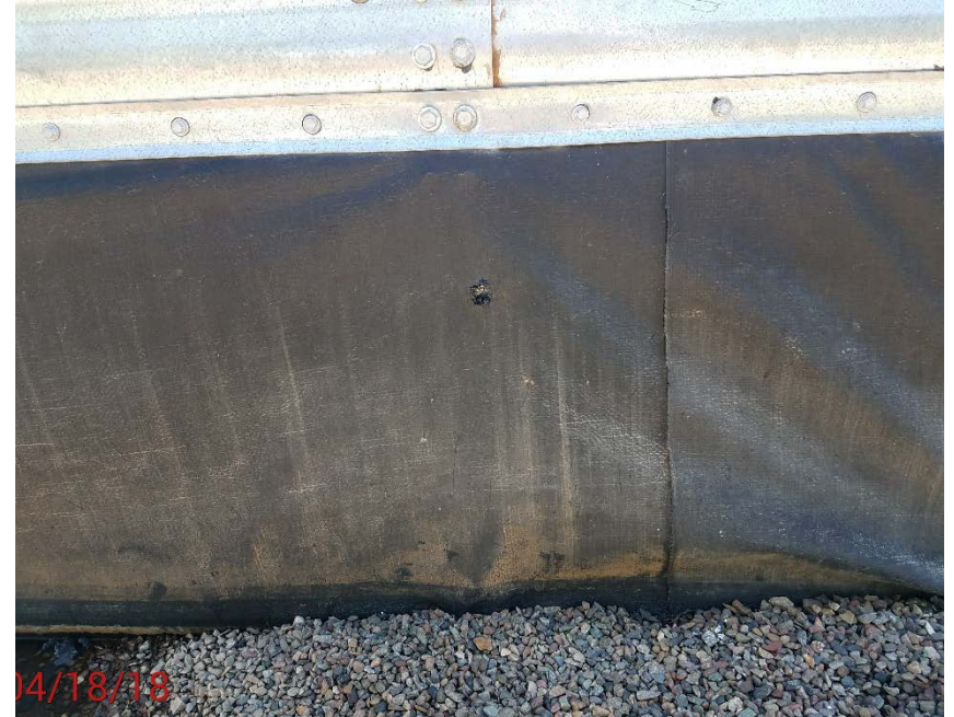
Location Photo # 2, hole in containment
