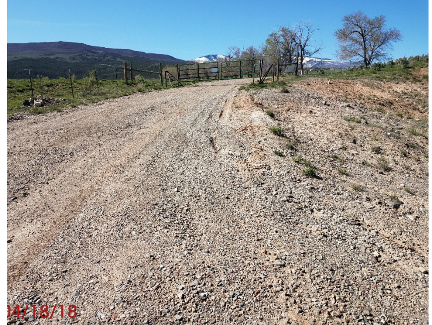
Location Photo # 10, storm water erosion
