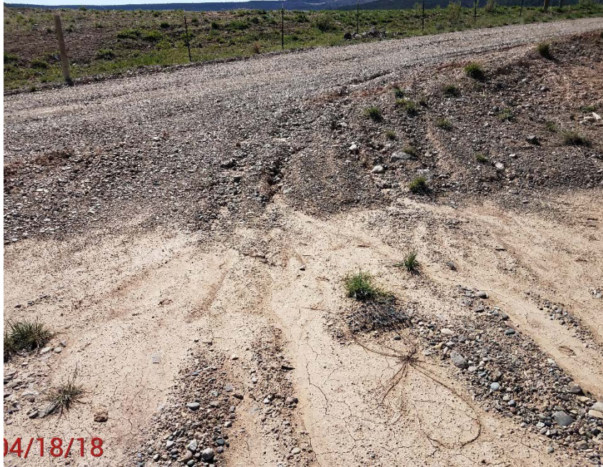
Location photo # 9, storm water erosion
