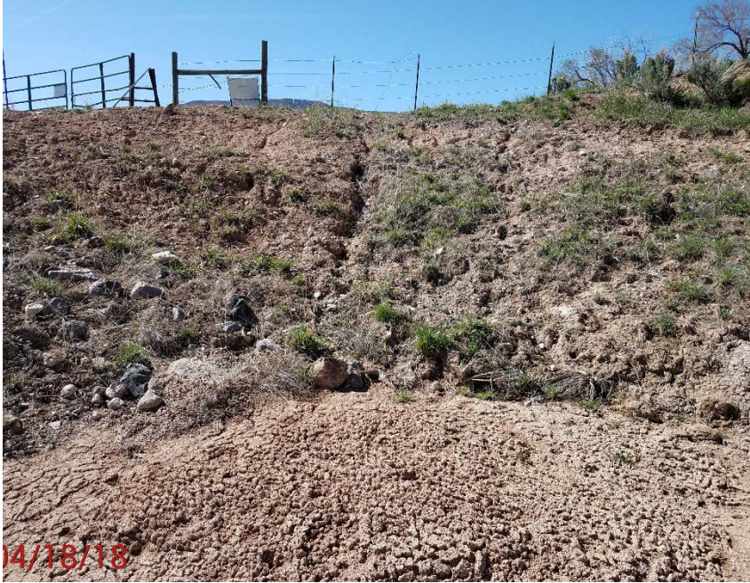
Location photo # 7, Storm water erosion
