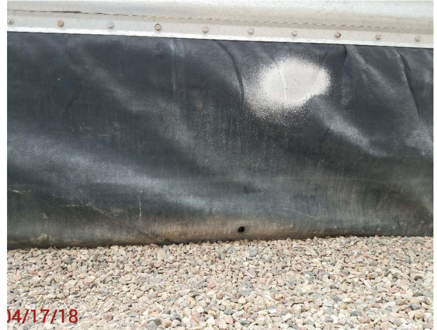
Location Photo # 6, Hole in containment
