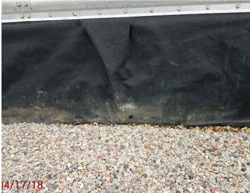
Location photo # 5, Hole in containment
