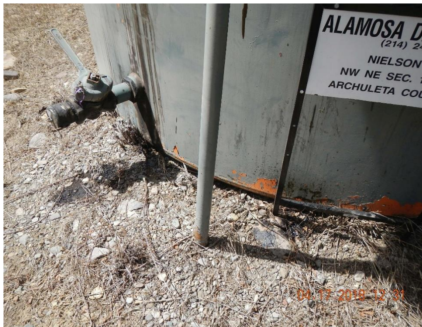
Stained soil beneath load out valve and below hammer union on flow line.
