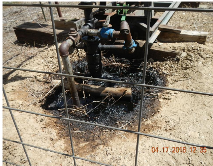
Oil stained well head and impacted soil.
