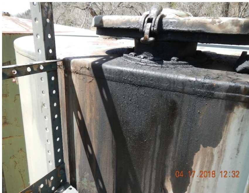
Oil staining on AST near thief hatch.
