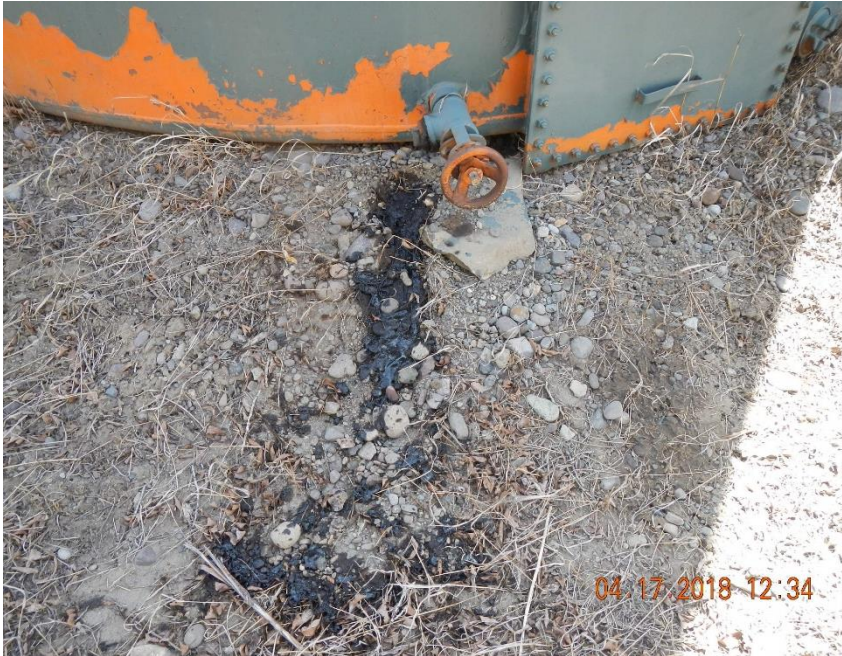
Stained soil beneath tank valve.
