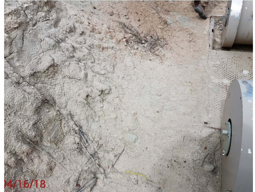
Location Photo # 16 slope erosion behind separators.
