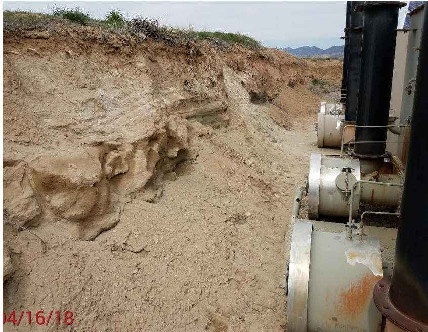
Location photo # 15, Slope erosion behind separators
