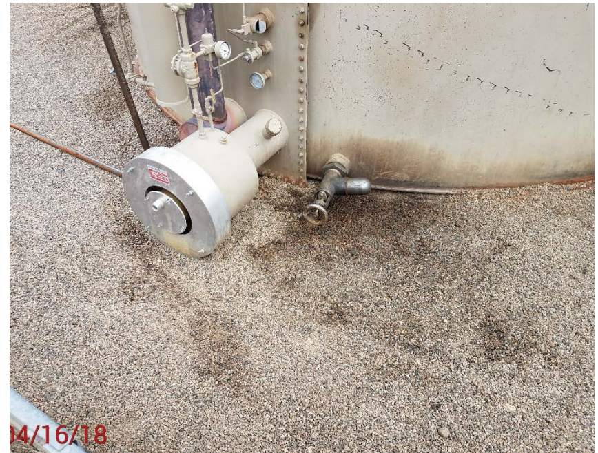
Location Photo # 14, leaking valve near heater unit in tank
