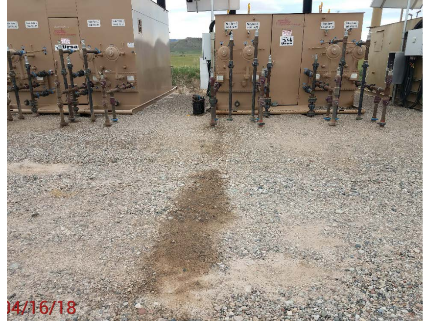
Location Photo #2 Stained soil by Separators
