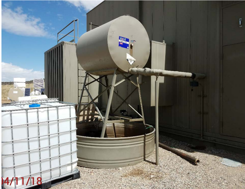
Photo # 11, Tank missing information. Unprotected container, netting missing
