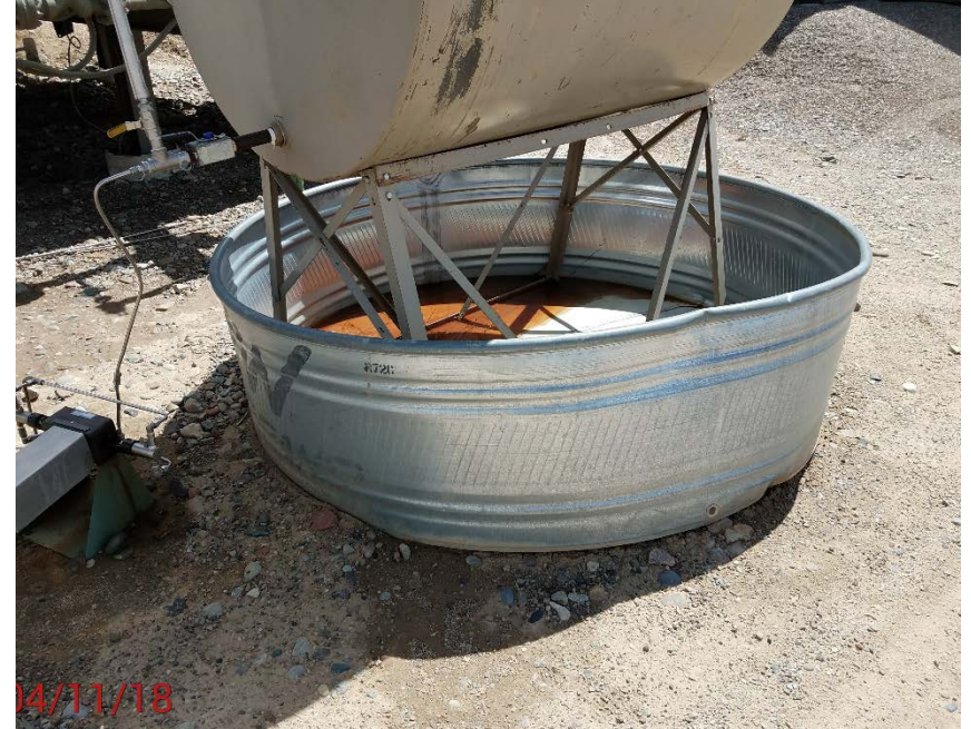
Photo # 8 unprotected container, netting missing.
