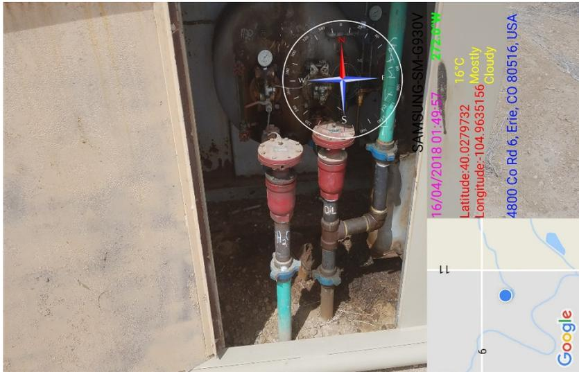
Leak and stained soil in dog house of separator
