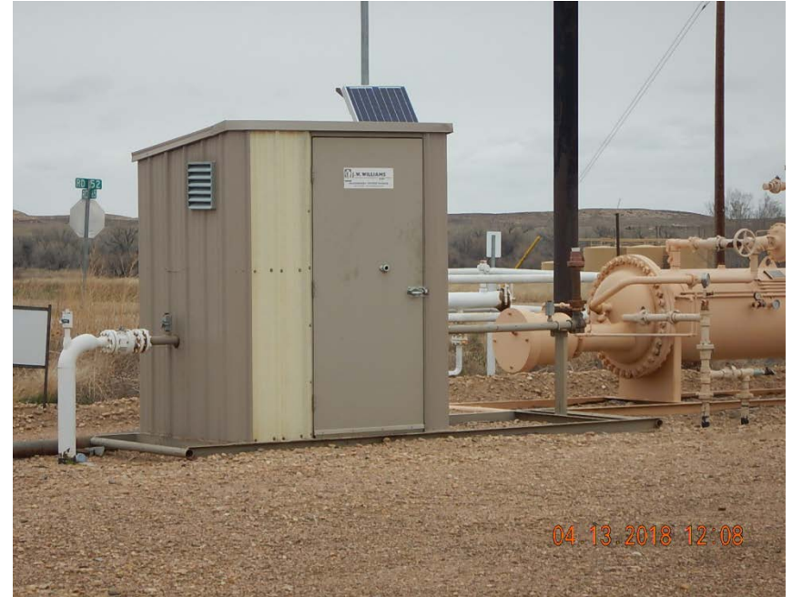
Photo 4: Unused meter run on location.
