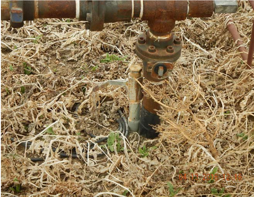
Photo 5: Unused flowline riser at wellhead.
