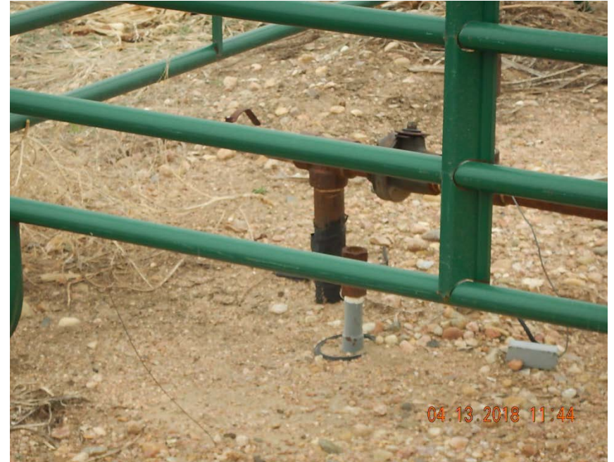
Photo 2: Flowline riser at wellhead.
