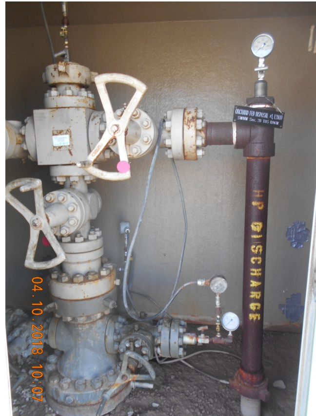
Wellhead inside housing
