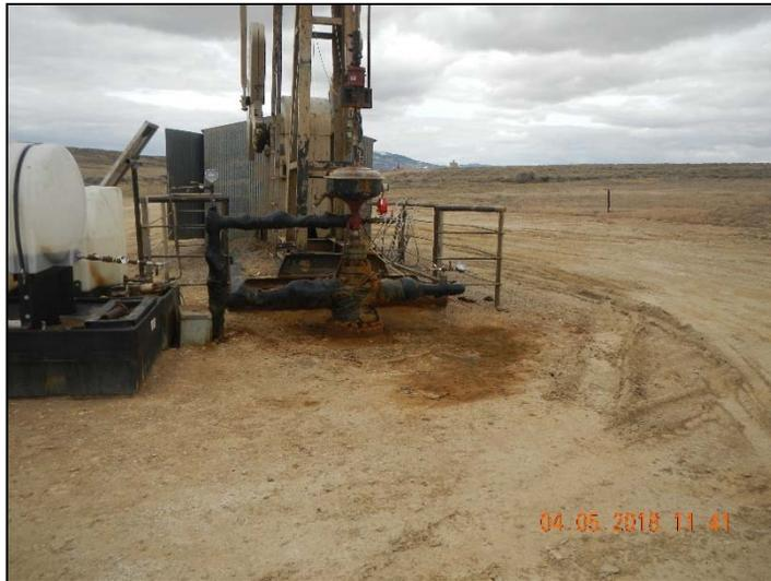
**Photo 3. Stained soil at wellhead.**
