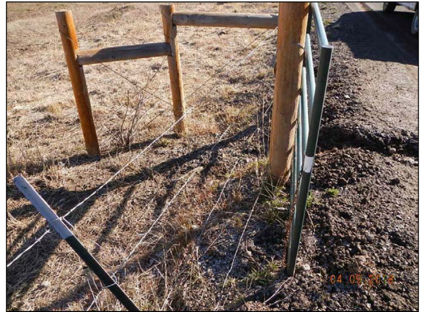
Photo 2. Erosion at gates with sediment migration into vegetation.
