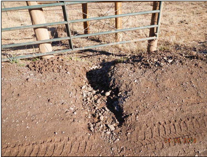
Photo 1. Erosion at gates with sediment migration into vegetation.
