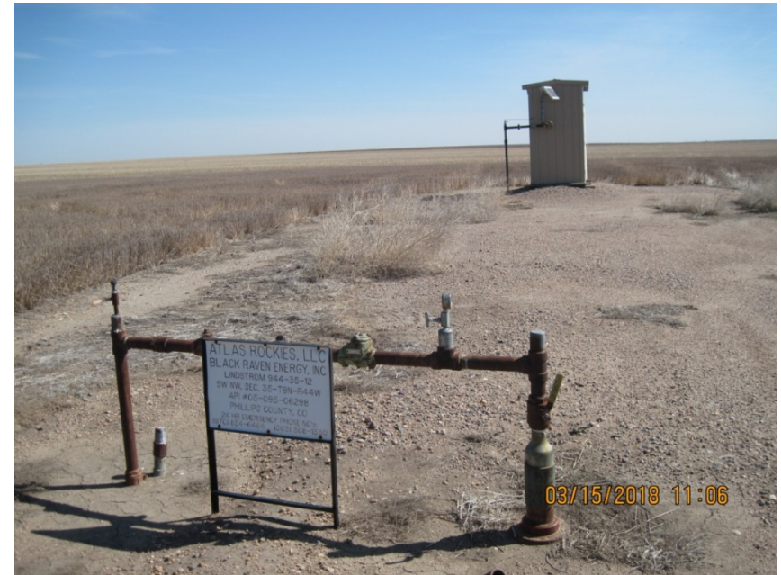
2. Wellhead and Meter shed
