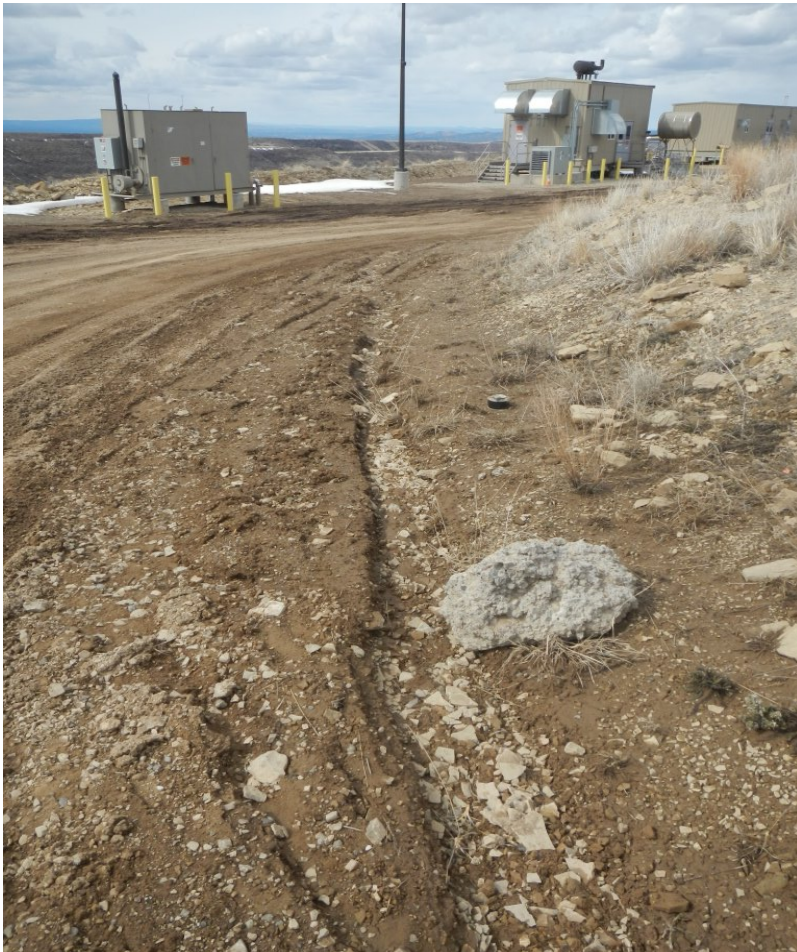
Photo#7: East side of Access road ditch needs maintenance.
