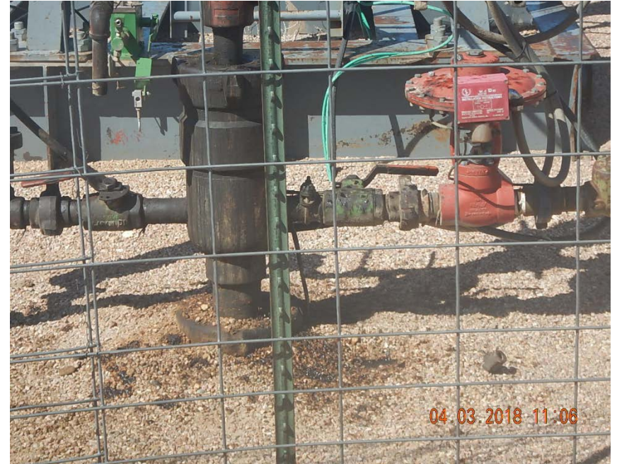
Photo 2: Stained soil at wellhead
