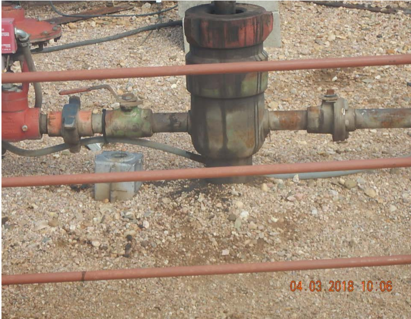
Photo 3: Stained soil at wellhead
