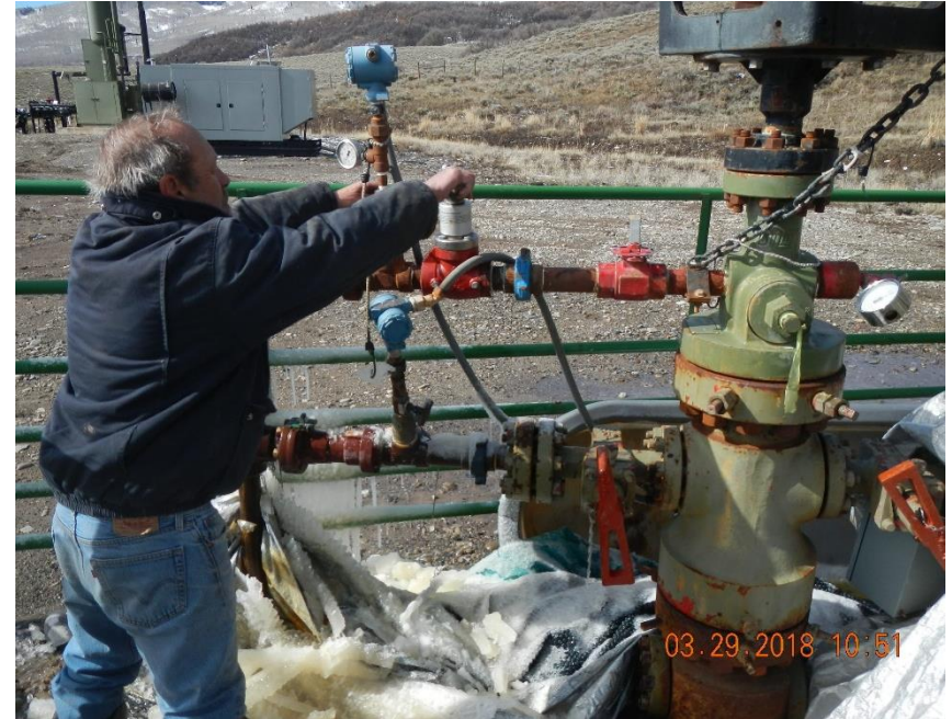
Gunnison Energy representative isolating release point.
