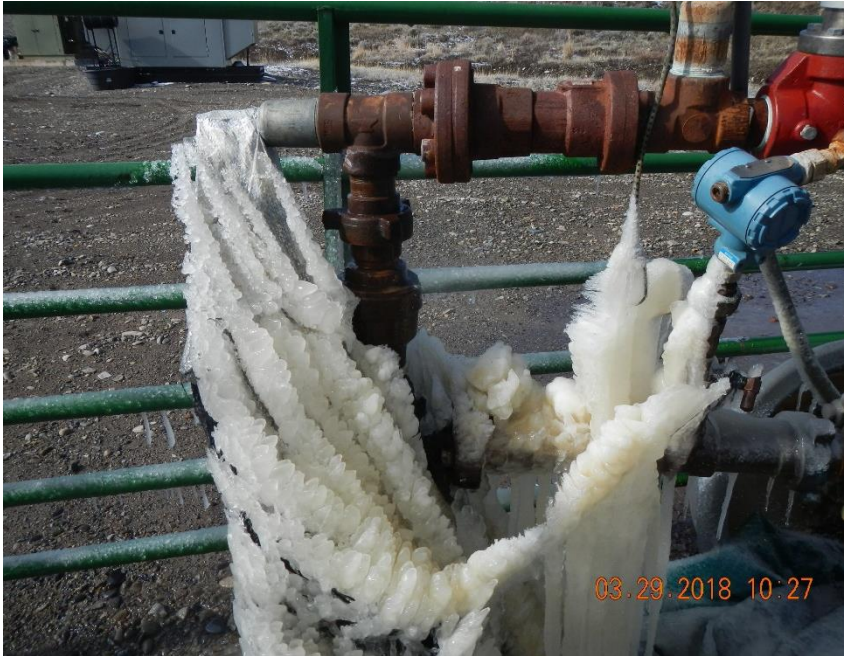
Leaking hammer union on production T.
