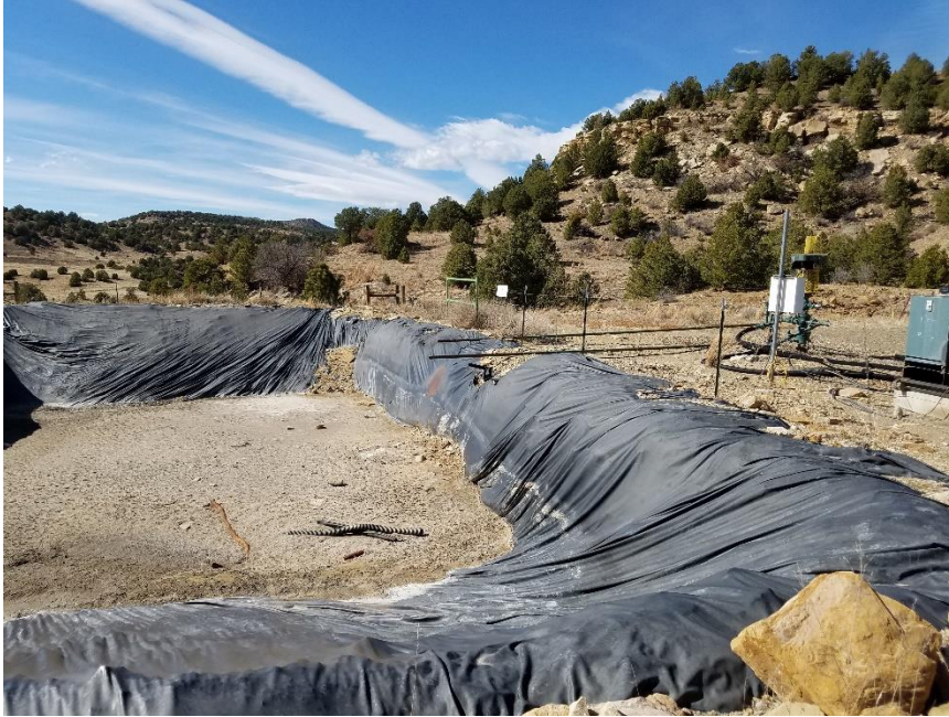
Photo 3. Holes in liner
