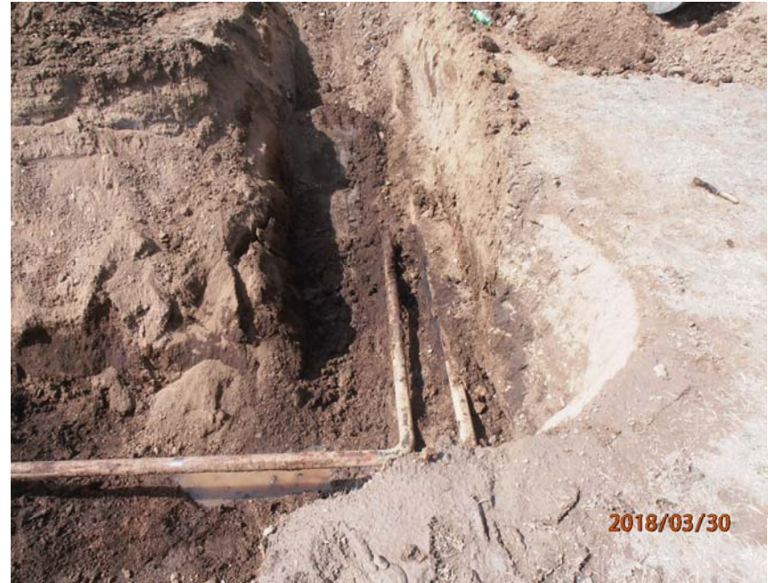
Photo 2 – Excavation at release area, looking west. Pipeline on right is apparently abandoned line from the plugged Priddy #1
