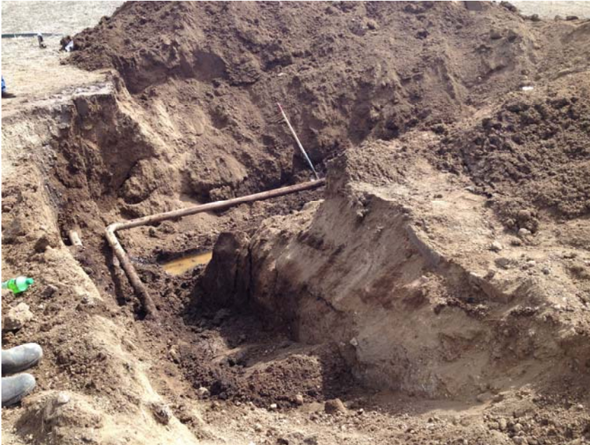
Photo 5 – Excavation at release looking approximately east-southeast. Impacted material remains in excavation.
