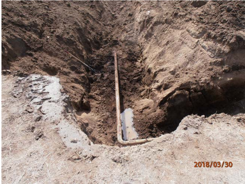
Photo 3 – Excavation at release looking south. Release was apparent at/near elbow in flowline.
