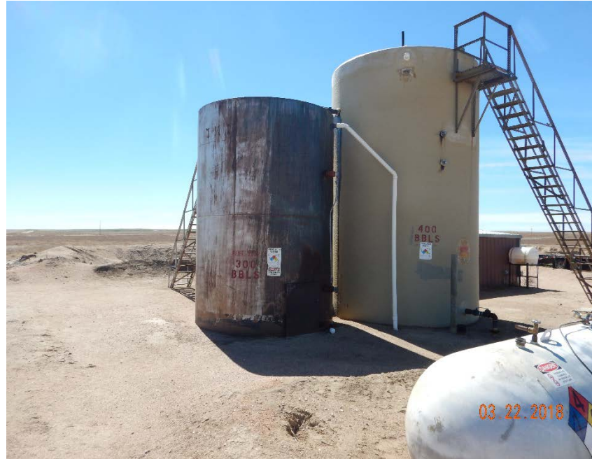
Photo #3 – Produced water steel ASTs. Note shallow earthen berms.
