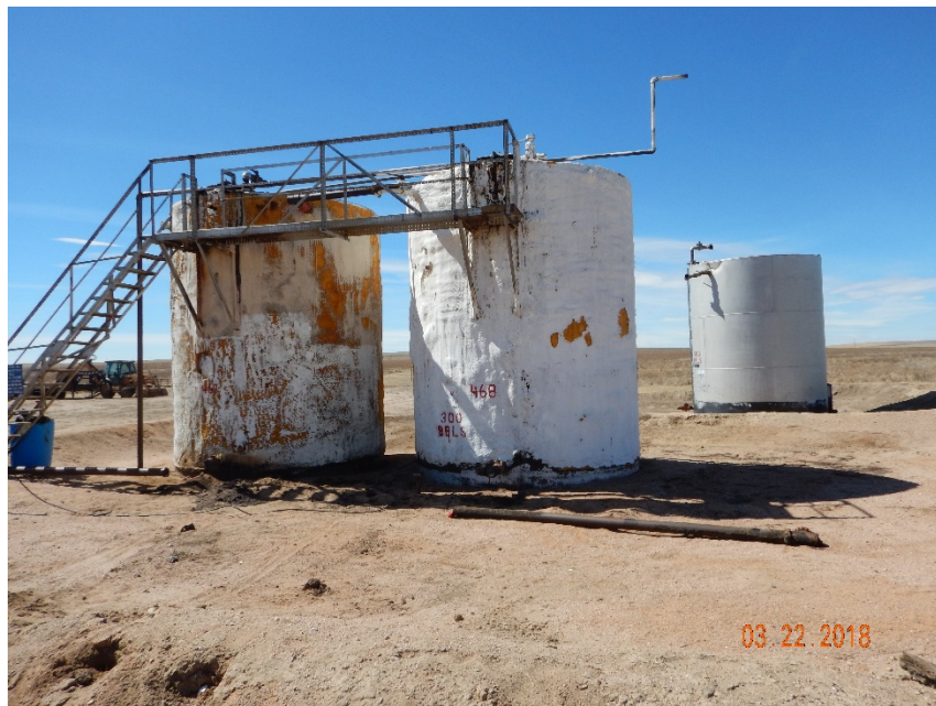
Photo #1 – Crude oil tank battery, looking west. Note eroded berms, lack of content labels, and damaged/faded NFPA placards.
