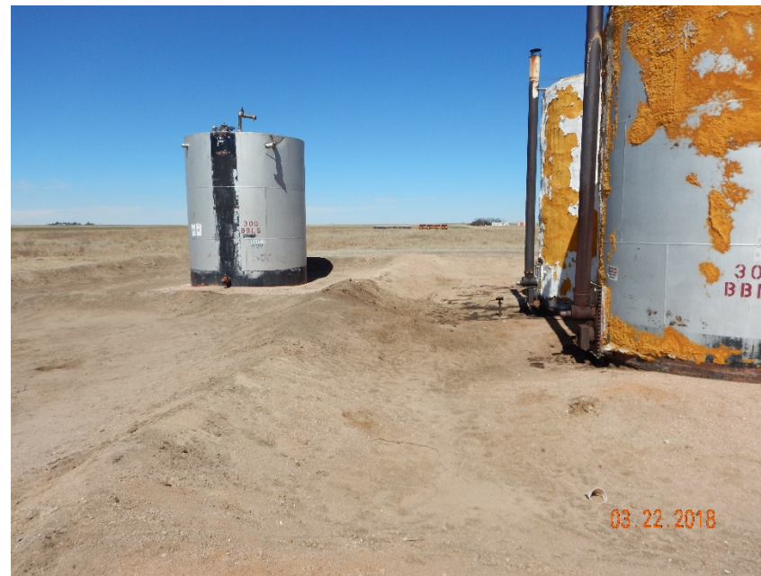
Photo #2 – Shallow earthen berms and oil-stained soil remaining between 300 bbl crude oil ASTs. Note west steel AST lacks content label and has conflicting NFPA placards (left side).
