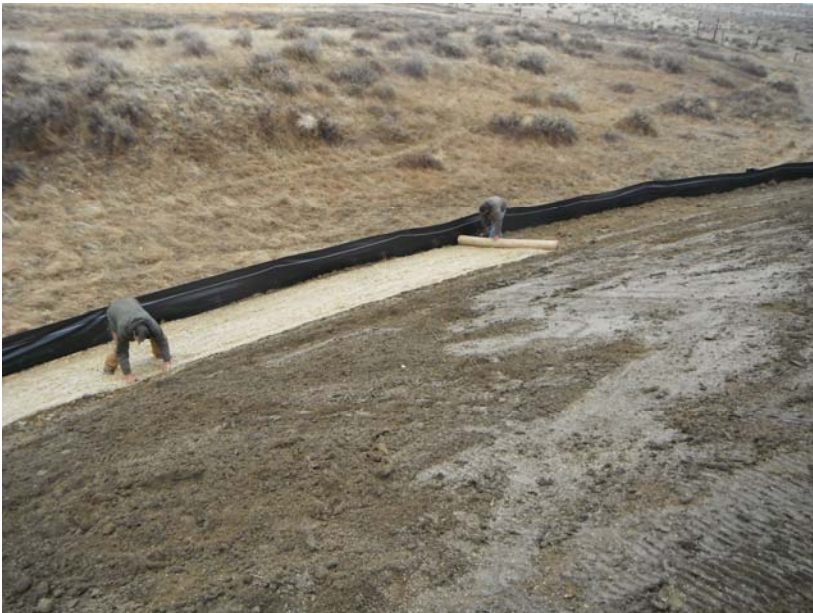
Installation of erosion control blankets
