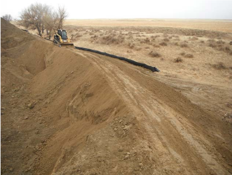
Creating flat surface on top of dike
