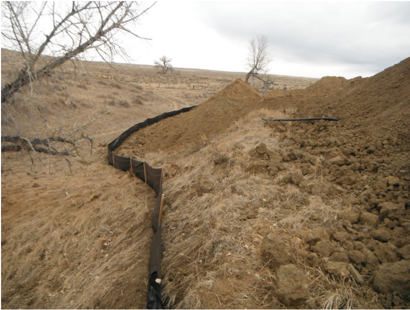
Silt fence installed on March 27
