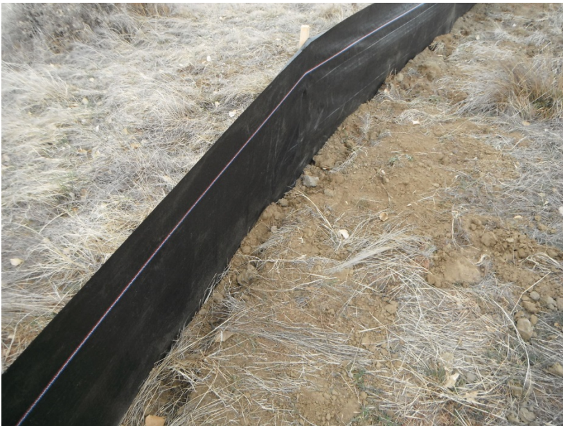
Silt fence detail
