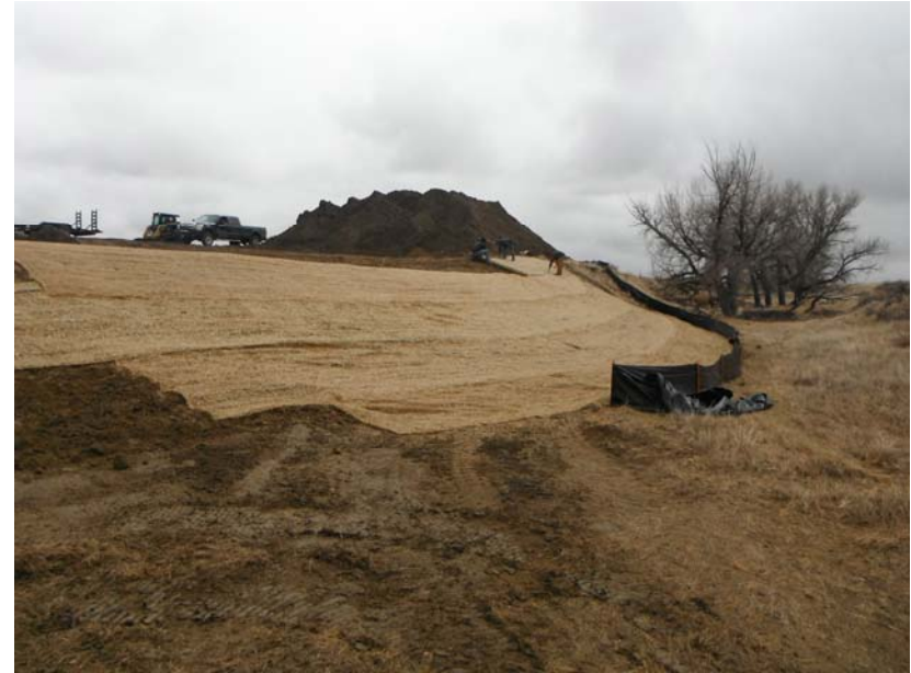
Installation of erosion control blankets
