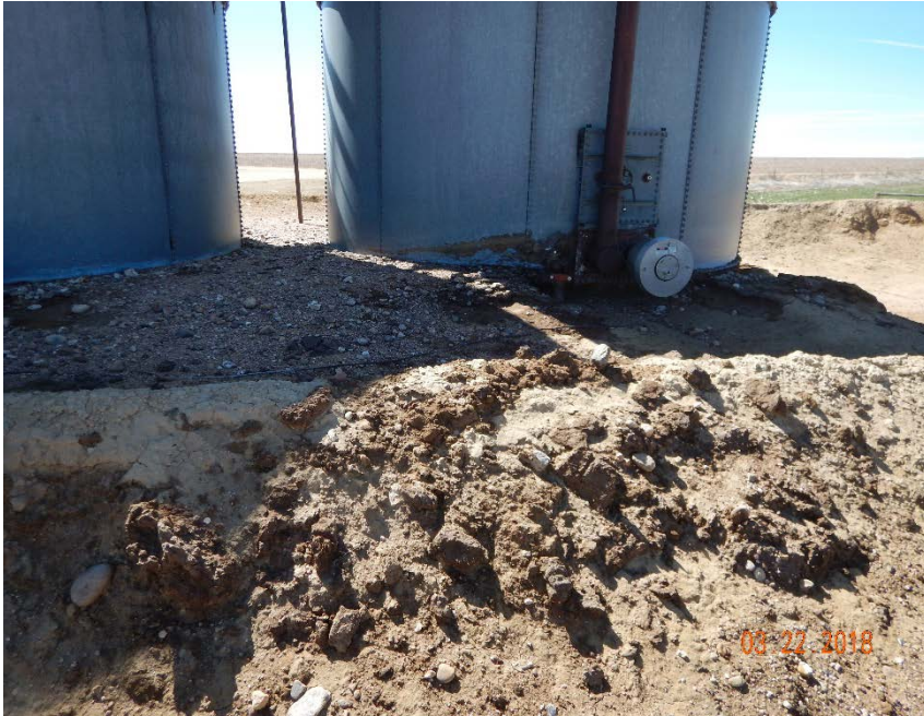
Photo #3 – Localized accumulations of oily waste and damaged berms on north side of crude oil ASTs.
