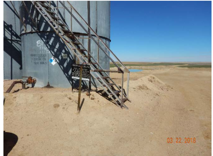
Photo #2 – View of 500 bbl crude oil ASTs from SE corner. Note shallow east berm.
