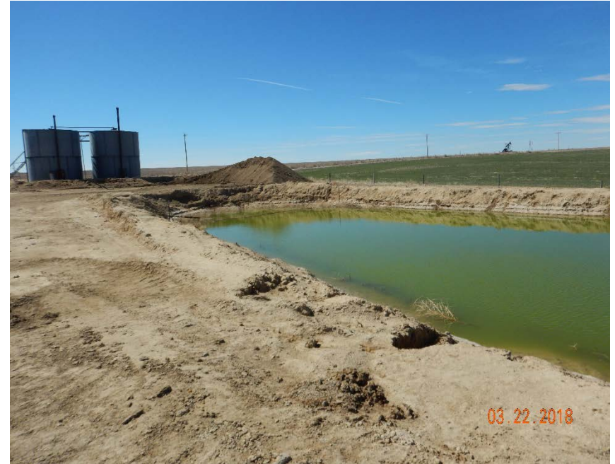
Photo #14 – West produced water pit has adequate freeboard.
