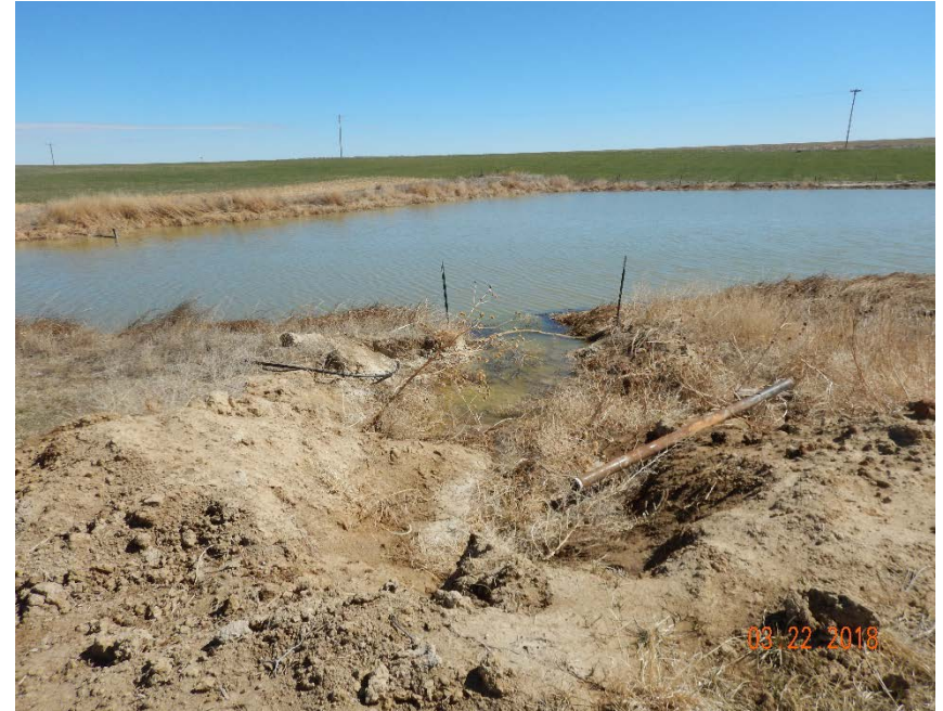
Photo #10 – Junk pipe located at NW corner of east pit. Note that pit lacks required 2' of freeboard and method of monitoring/maintaining freeboard required by Rule 902.b.
