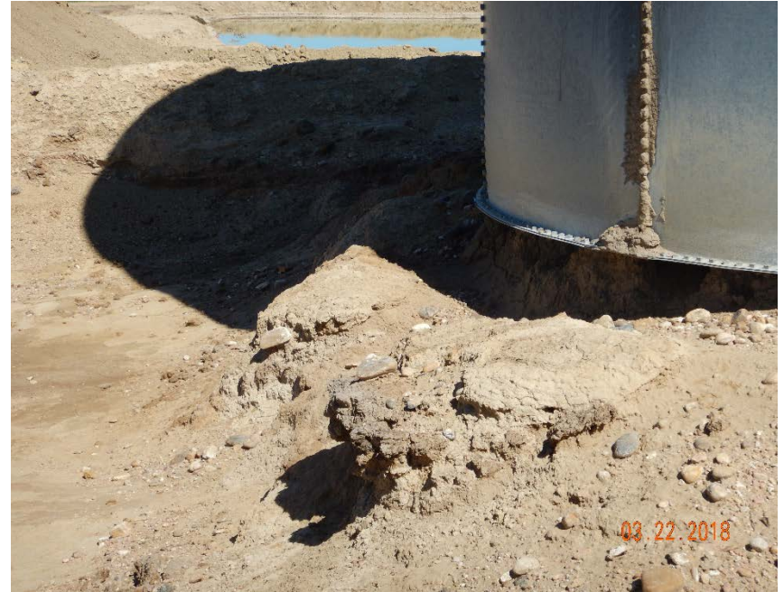
Photo #4 – Historical accumulation of oily waste and erosion of base of earthen berm on west side of crude oil ASTs.
