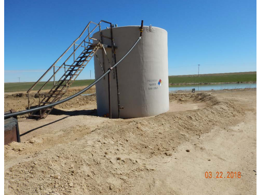
Photo #6 – 500 bbl produced water AST located on north side of tank battery (view from west). Note shallow earthen berms.
