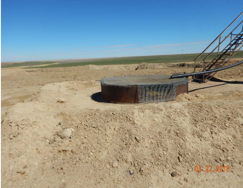
Photo #7 – View of skim tank on north side of tank battery. Note shallow earthen berms and absence of required NFPA placard as well as volume/content labels.
