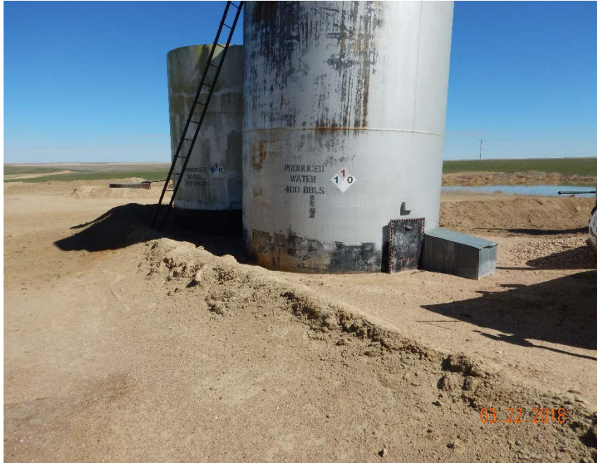
Photo #9 – View of shallow earthen berm shared by 200 bbl and 400 bbl produced water ASTs on east side of tank battery.
