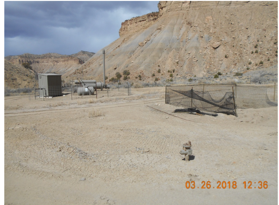
Unused riser , blowdown pit with damaged netting,
