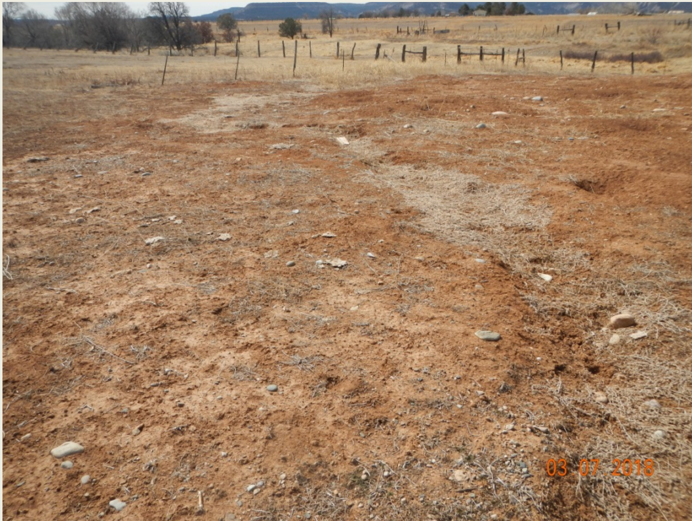
Photo 4. View of drainage area where erosion is occurring in the south-central portion of the project area. Stormwater controls are needed.
