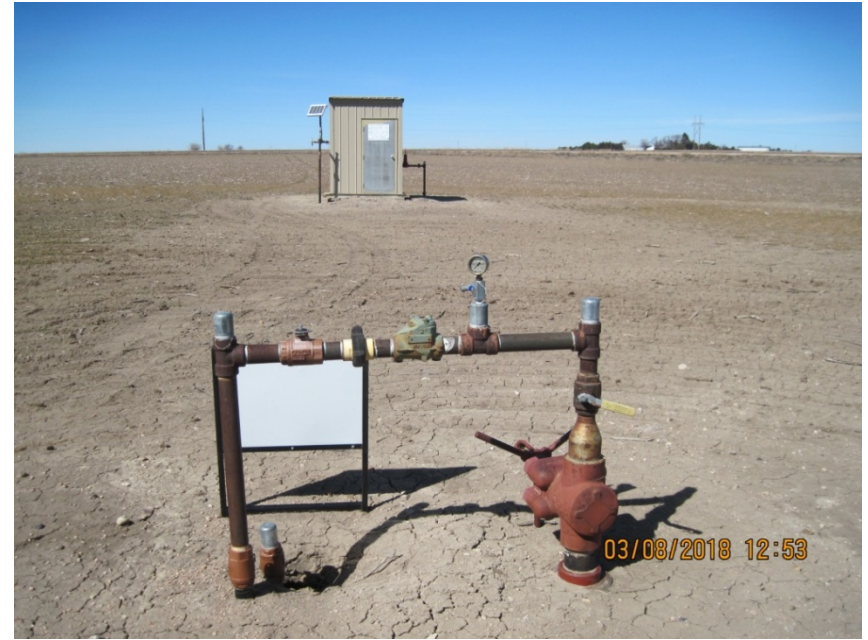
2. Wellhead & Meter shed
