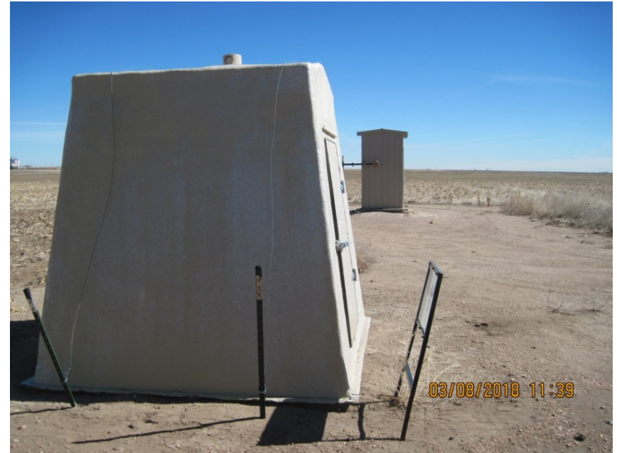
2. Meter shed & Wellhead covered with fiberglass shed
