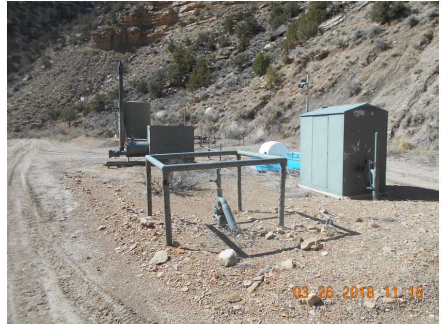
Separator and Meter housing. Flowline riser.
