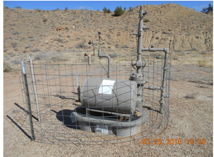
Wellhead and chemical drum. Label on drum illegible.
