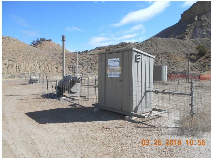
Separator and Meter housing with sign
