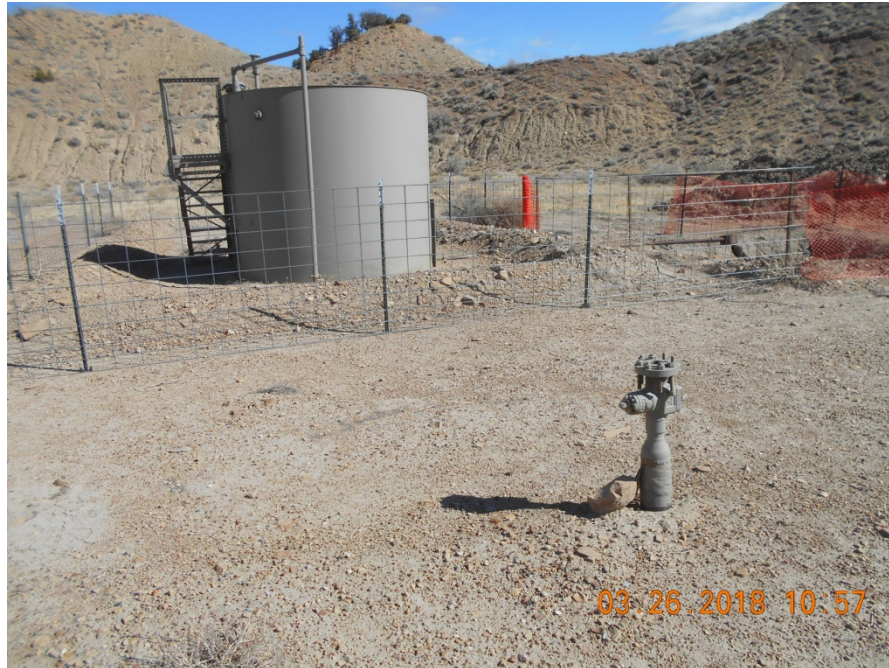
Tank Battery with unused flowline riser.
