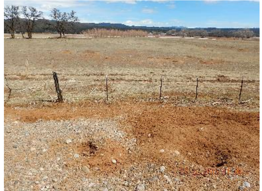
Photo 4: Animal burrows and drainage erosion channels in E fill slope.
