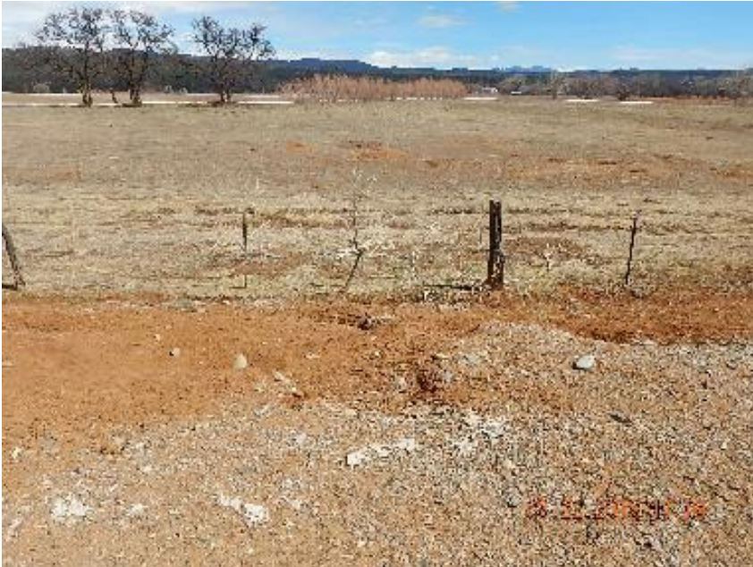
Photo 3: Animal burrows and erosion drainage channels in E fill slope.
