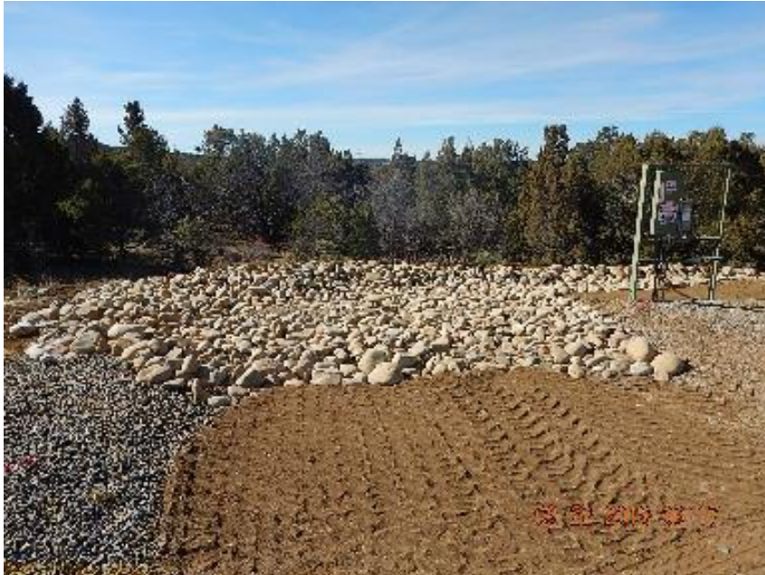
Photo 5: Repaired area at top of fill slope.
