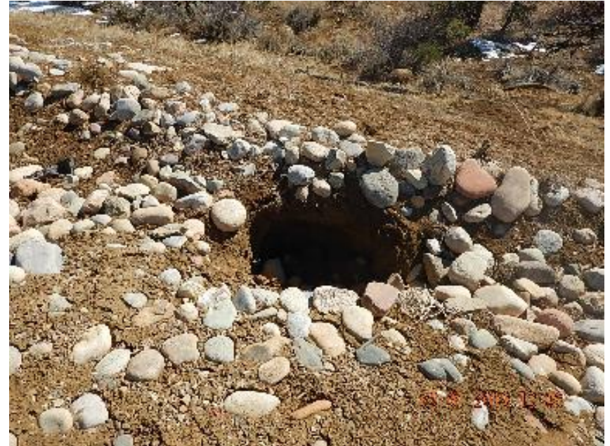
Photo 4: Sink hole at top of S fill slope previous inspection.
