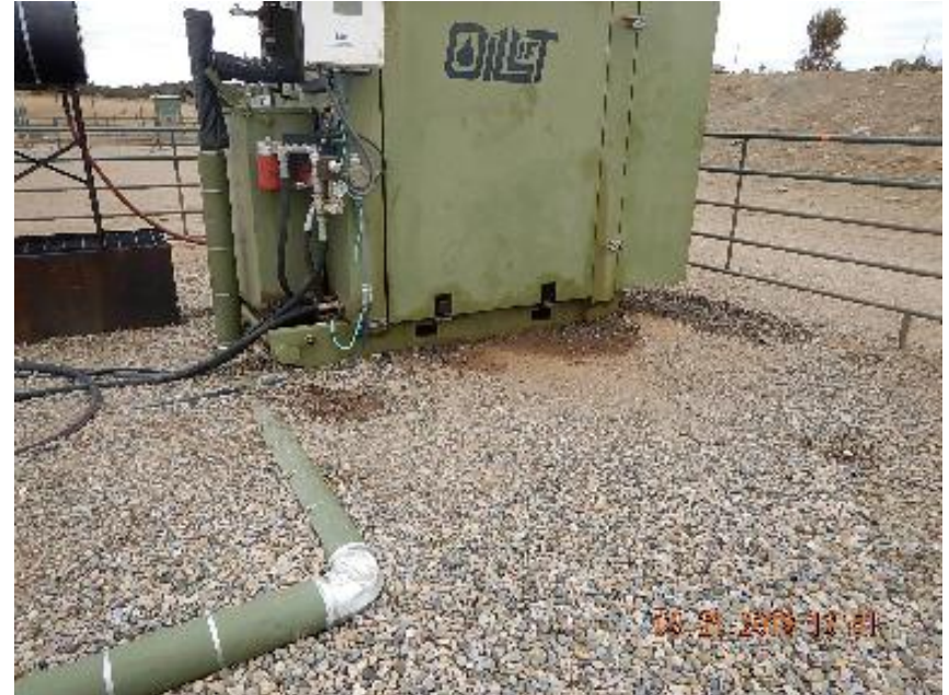
Photo 6: Impacted soil and gravel around base of oil lift unit.
